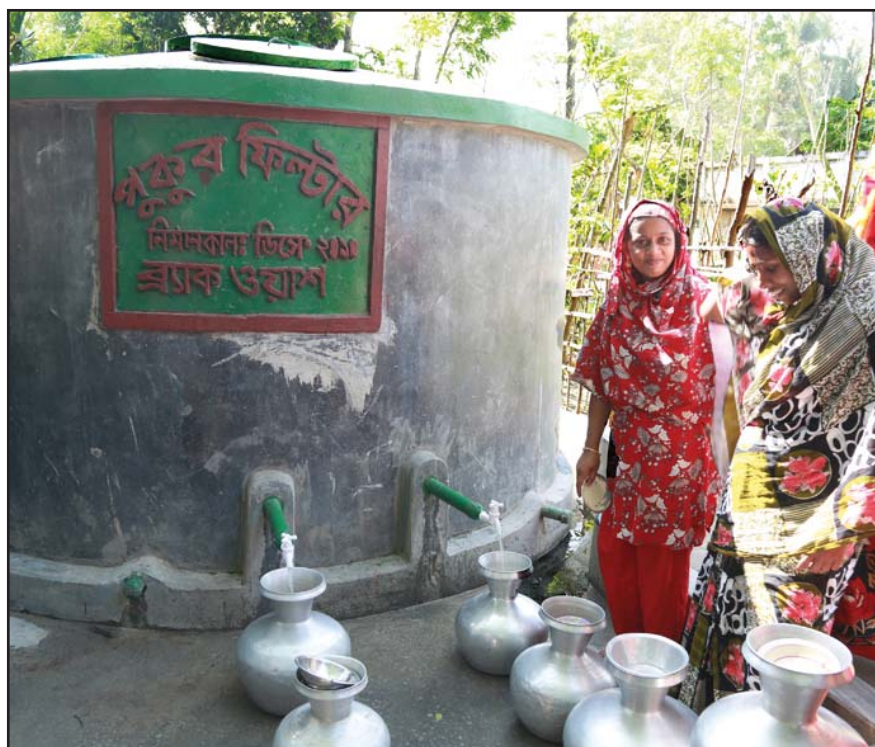
Collecting water piped from a pond sand filter at Barobaria village in Bagerhat.
