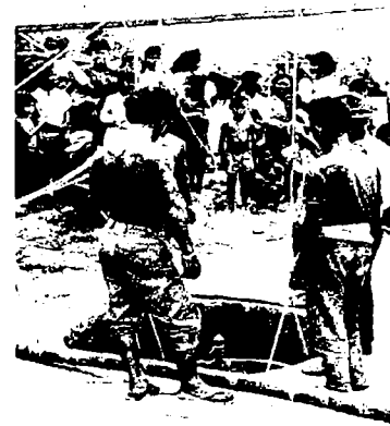
Installation of a hand-dug well in Cambodia is part of the Community Self-Improvement (COSI) programme in that country.
