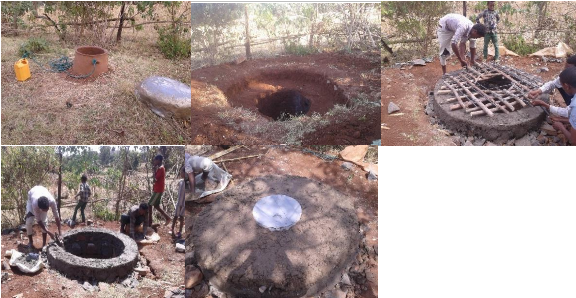
Figure 6 Improved well head of Minalu Alehegn (Debre Yacob)
