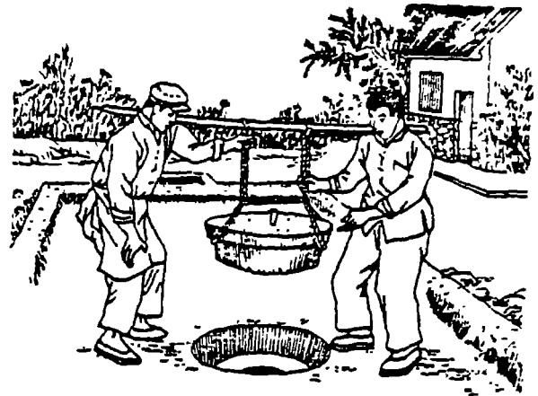
Fig. 4-23. Fitting a removable cover.
