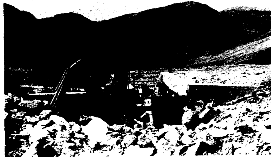
Fig. 1.3 Storm damage to Noe intake
