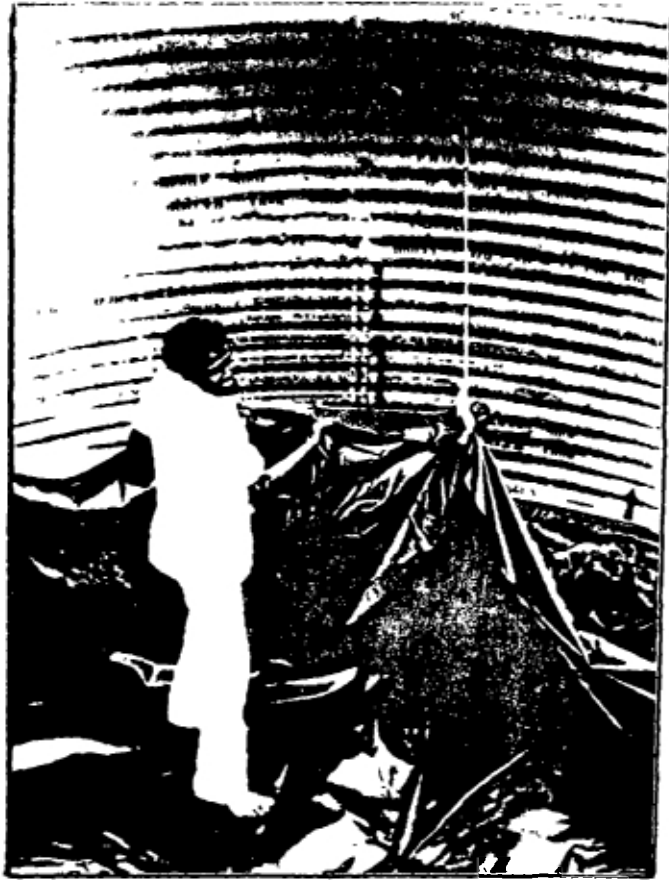
Fig. 15 Liner being Fitted into a Raw Water Tank
