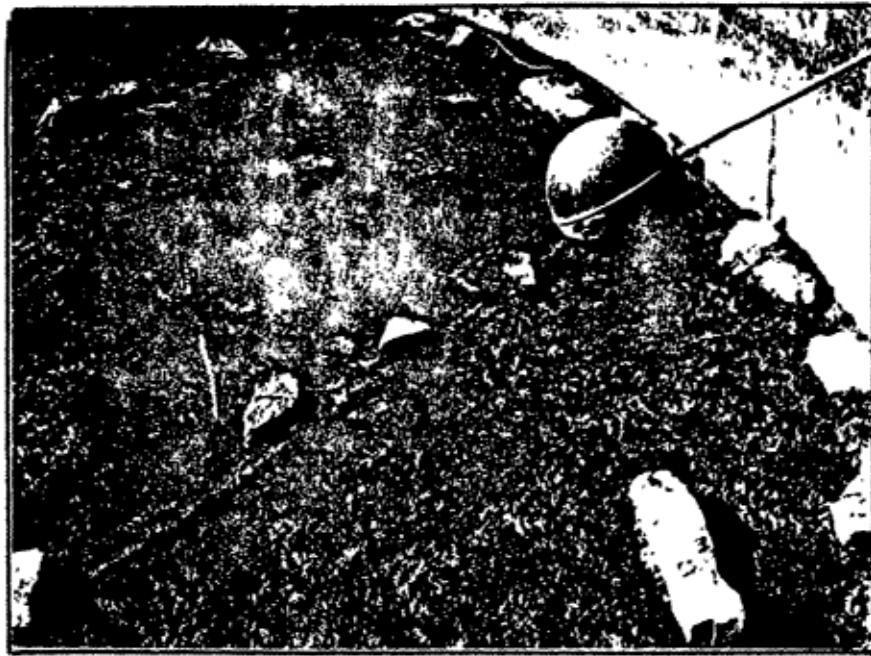
Fig. 22 These Filter Mats have to be Cleaned
