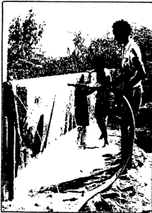
Fig. 23 Cleaning the Filter Mats
