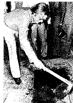
Mr. G.H. Read (in the fore front) Sanitary Engineer from the Ross Institute of Tropical Hygiene, London, excavating the dry digested sludge from the twin-pit of a Sulabh Shauchalaya at Patna.
