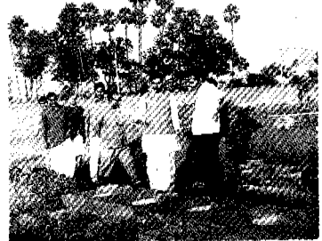
Mr. V.S. Dubey, District Magistrate, Patna, visiting the construction site of temporary Sulabh Shauchalayas during a conference at Patna.
