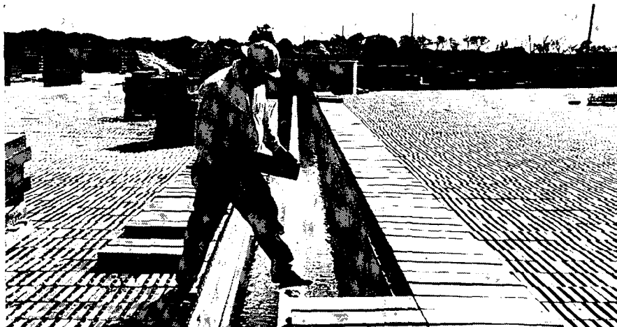
■ CHANNEL block made by Can-Tex Industries being placed in one of the filters which serves the Central Sewage System of the Trinity Valley Authority near Dallas.
