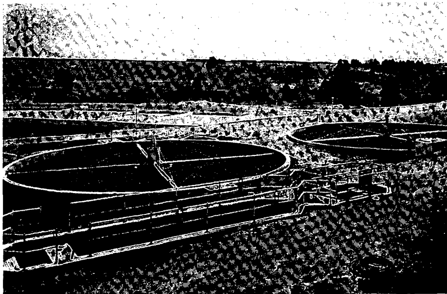
■ DISTRIBUTOR with multiple arms is a feature of the Aero-filter in a Gaffney, S. C. installation. Below are shown the secondary units of a two-stage filter plant that provides treatment for the Air Force Academy.
