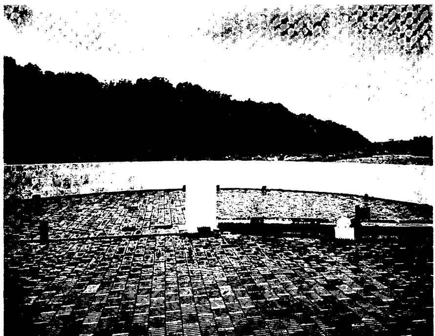
■ DICKEY high-rate blocks were used in the trickling filter at Springdale, Ark.
