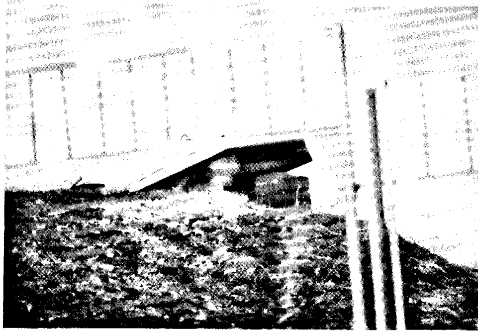
14. Broken vent on large city reservoir, Yerevan
