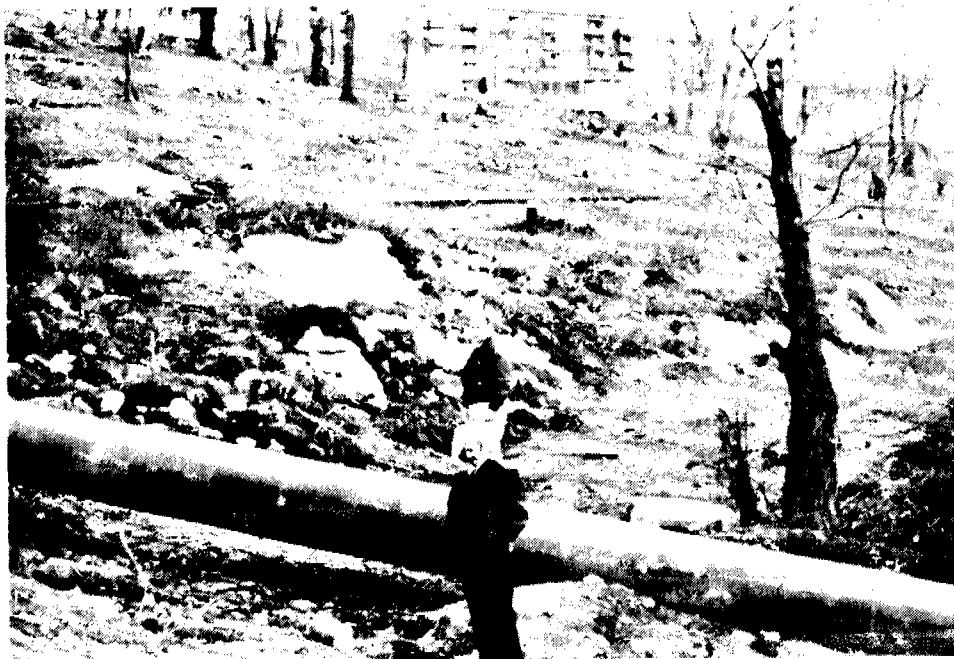
18. Sewage cascading down hill side (at feet of Suzanne Olds, U.S.AID/Yerevan Mission Head)
