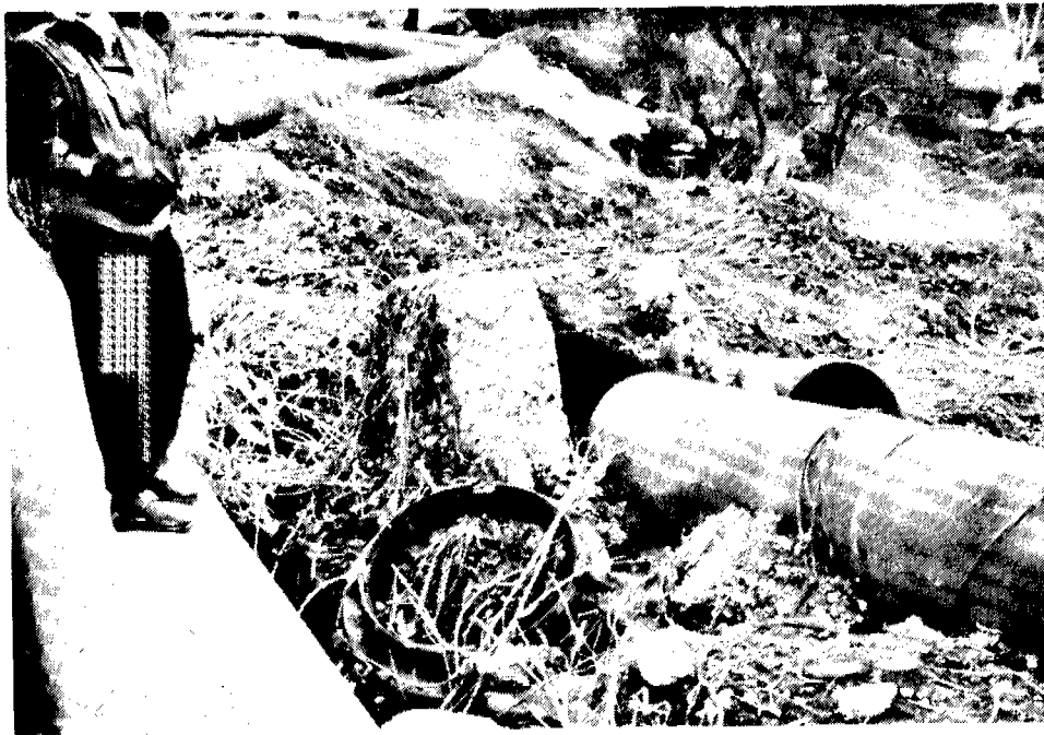
19. Broken sewer liner near "Massive"
