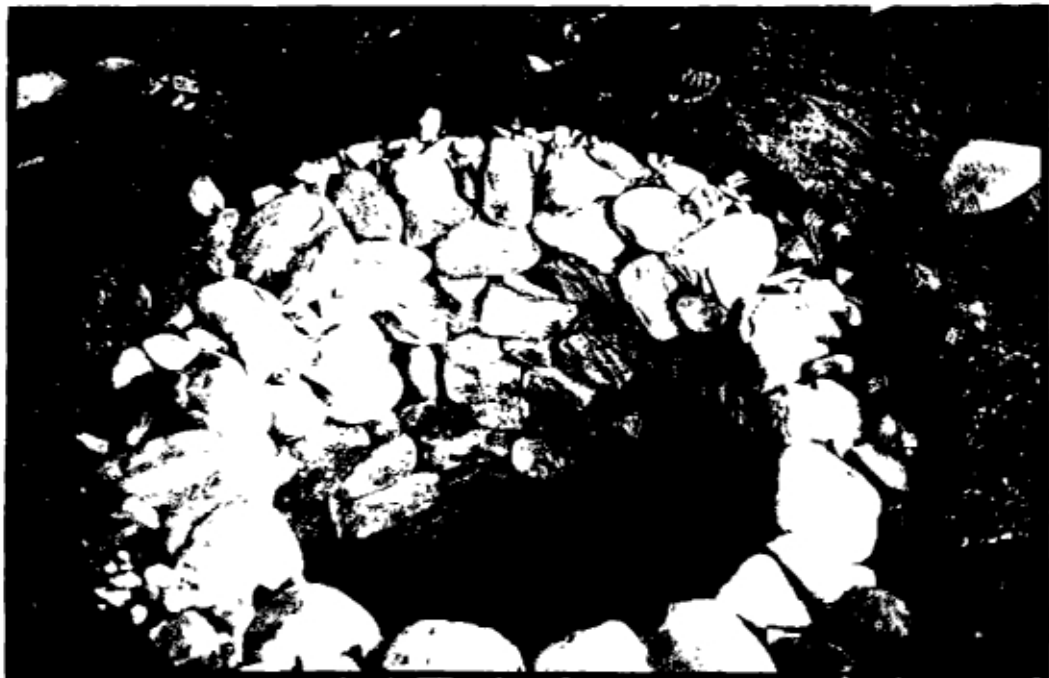
131. Also the pits can be made with local materials at low cost as shown here.
