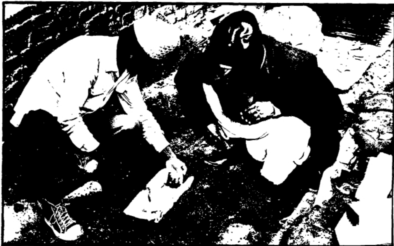
122. A mould made of timber or concrete is used to press the shape of the water seal into the ground.
