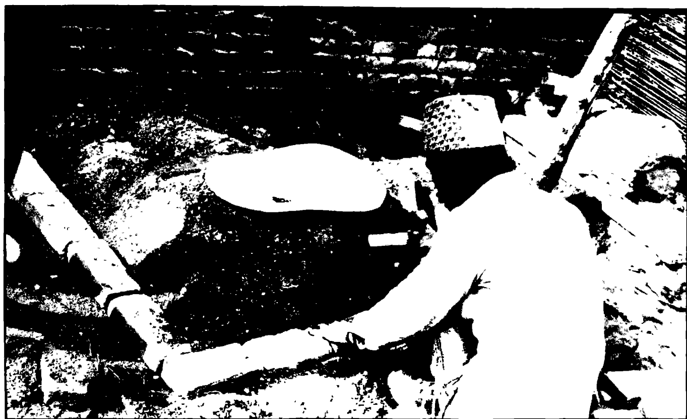
127. Dry bricks are used to build the soil platform around the pan.
