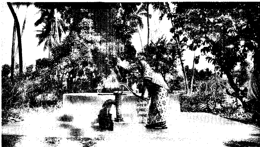
Sanitary well and hand pump at Totapalli village, block Chatarpur
