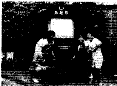
Photo 2-1 “ROJISON”, Water Tank Installed on a Street
