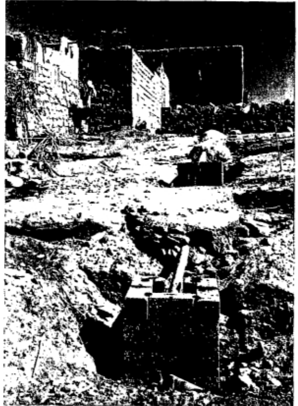
Tertiary sewers in rocky area
