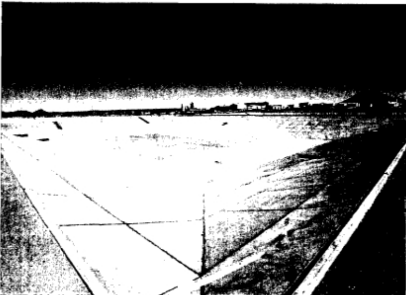
Anaerobic pond, empty
