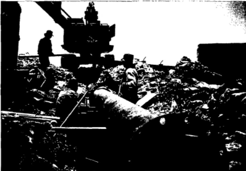
Transmission main between NWSA compound and storage reservoir:
