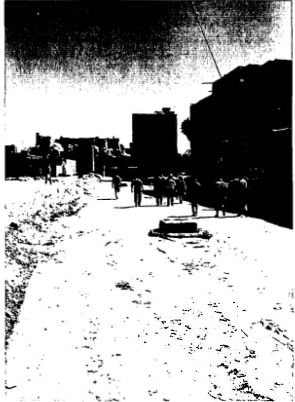
Graded road, with manhole up to future pavement level
