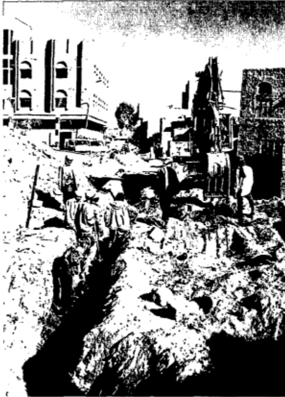
Digging trenches for sewer pipes
