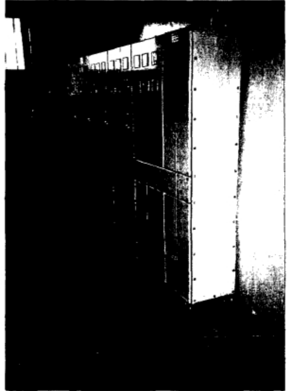
Control panels for generator sets
