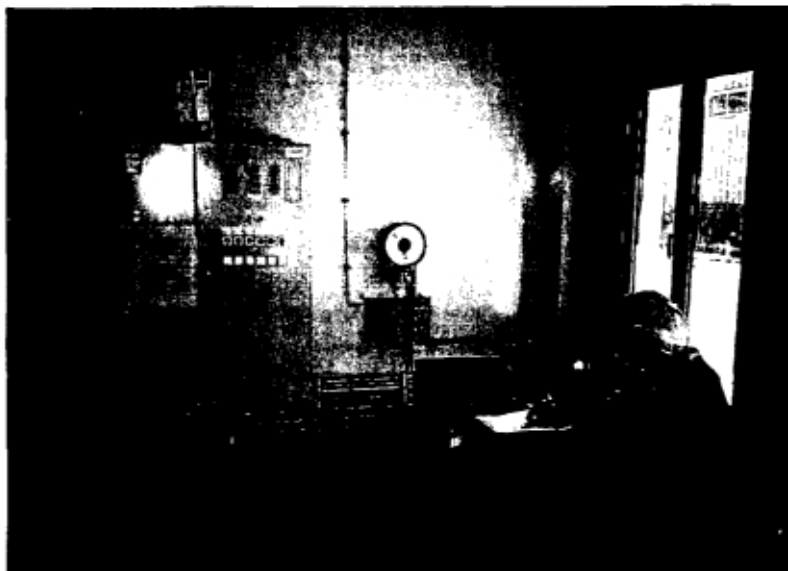
Main control centre with operating panel and reservoir water level indicator at back
