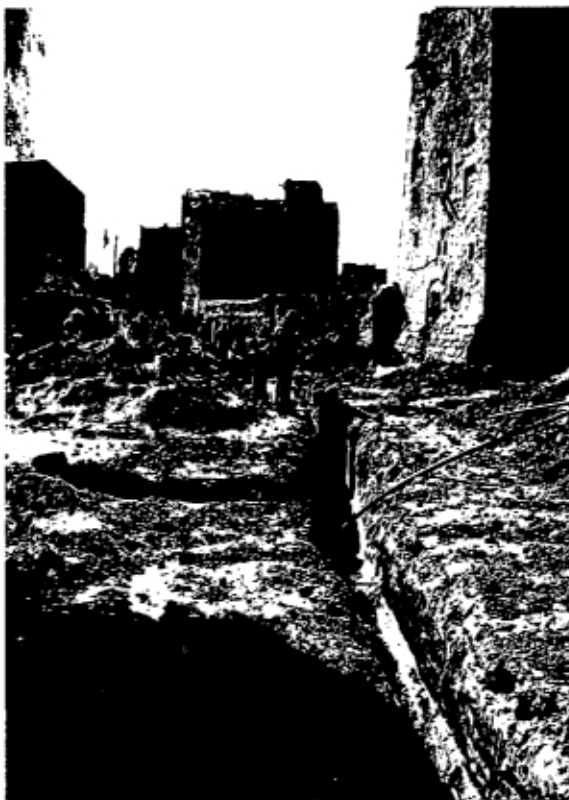
Excavation of trench for distribution pipes
