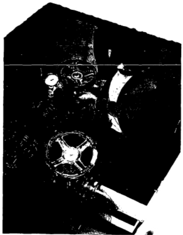
Opening flow to a district and checking the pressure
