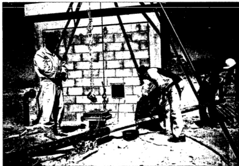
Submersible pump and riser pipe assembled, ready for lowering in borehole
