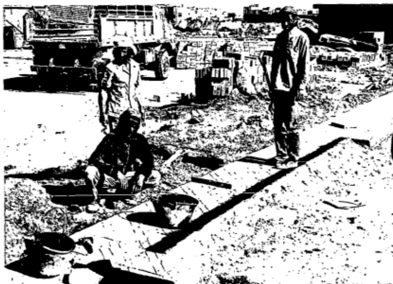
Placing kerb stones (top) and laying concrete tiles for sidewalks (bottom)
