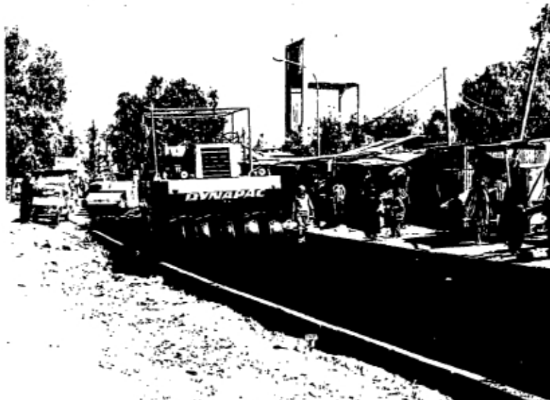
Surface drainage works: applying tack coat (top); laying binder course (centre); compacting binder course (bottom)
