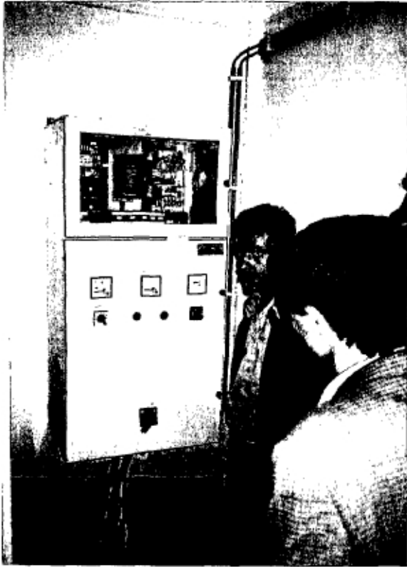
Switch panel inside pump house
