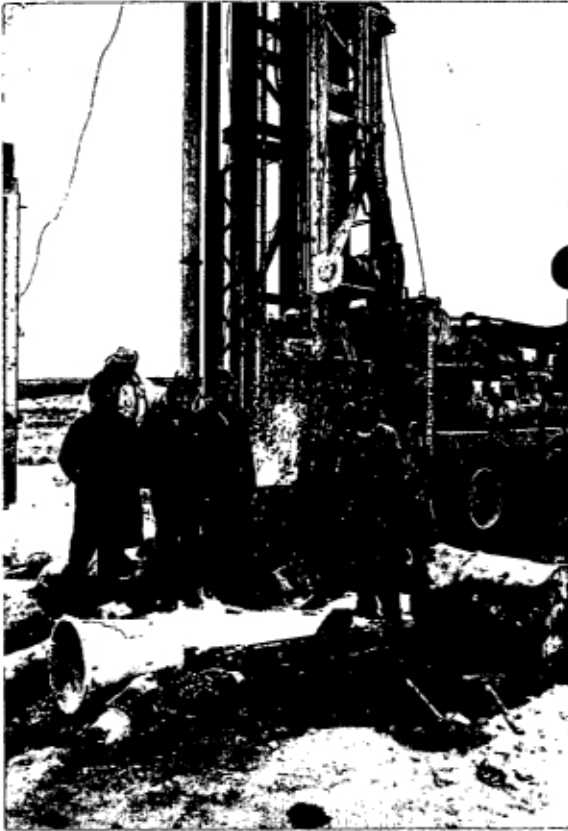
Drilling rig and crew on site
