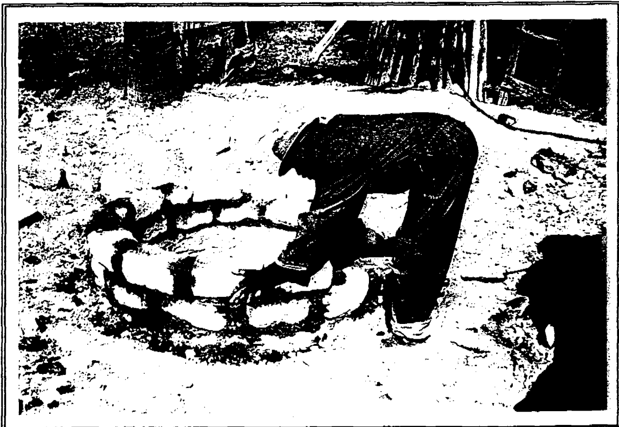
LOCAL LATRINE UNDER CONSTRUCTION
