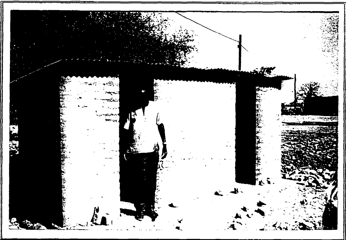
FOUR UNIT SCHOOL LATRINE UNDER CONSTRUCTION IN OKATOPE
