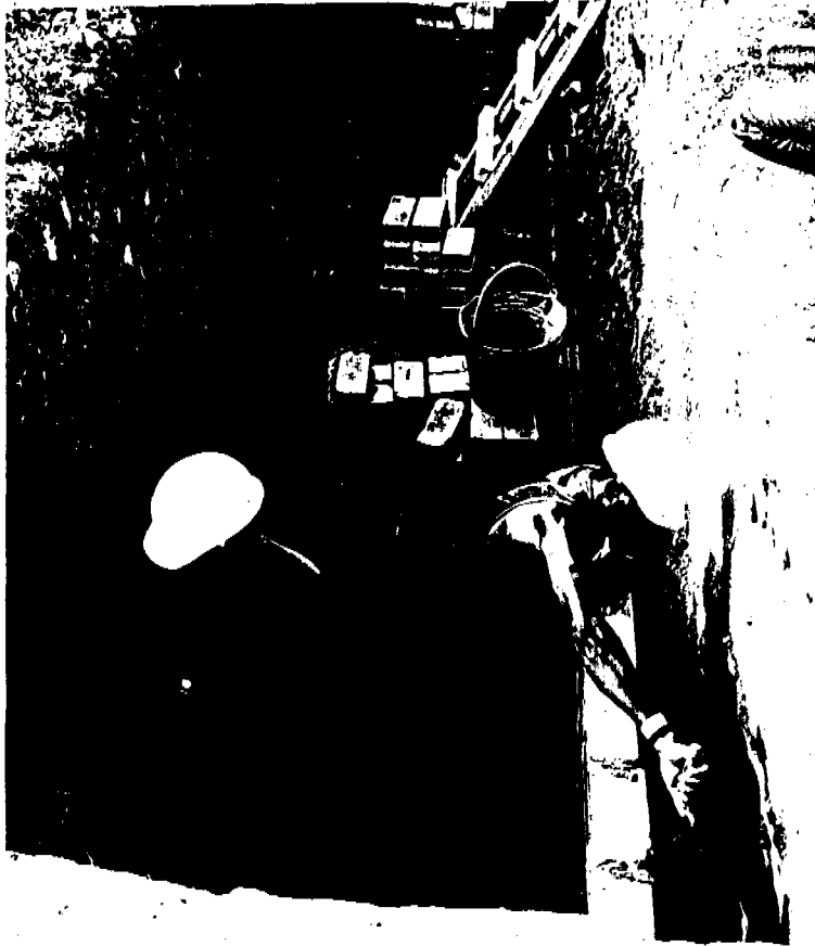
Bricklaying in the pit.
