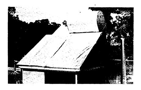
Figure 2: Tubing-type Solar Water Heater
