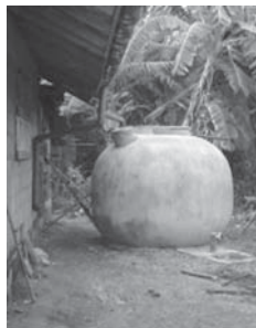
Ferro cement above ground tank
