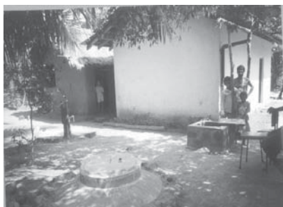
Brick under ground tank
