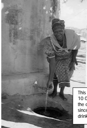
This Ferro cement tank holds 10 000 litres of rainwater, and the owner has been using it since the drought of 1993 for drinking and cooking.
