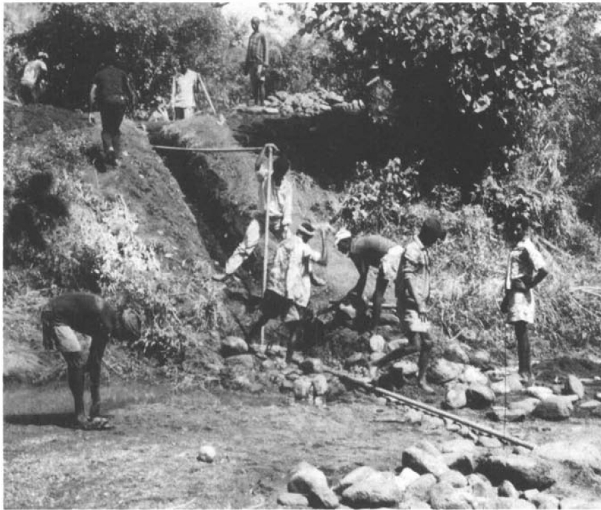
A sandwell under construction. Note the sealed well at bottom right.
