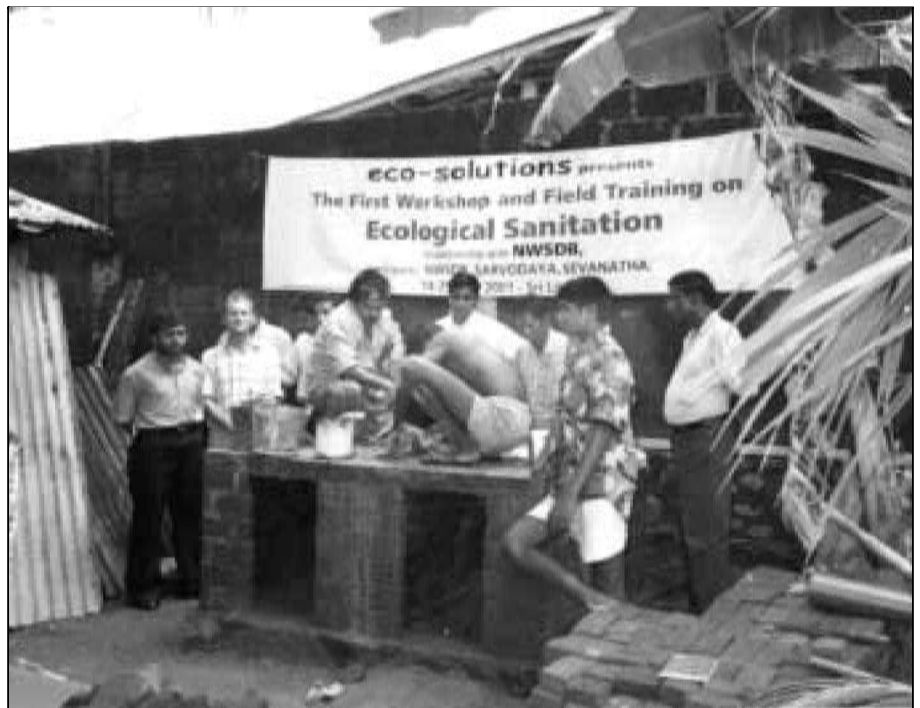
A toilet under construction during the training programme
