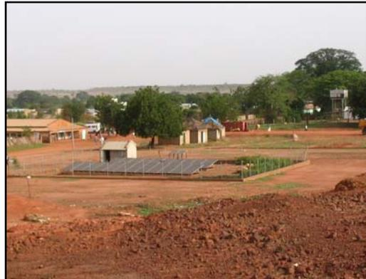
2. Increasing cell efficiencies (up to 16% achieved with Kyocera polycrystalline silicon solar panels where previously it was 5-6%) and new cell materials and manufacturing processes promise to bring the capital costs of solar powered schemes down significantly over the next decade. Such a lowering of costs brings solar-water pumping within reach of poorer communities.
