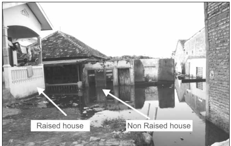
Raised and non-raised houses in a coastal area of Semarang
