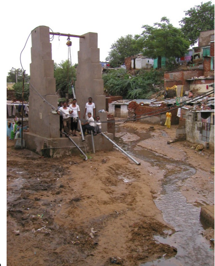
Above: Borewell maintenance
