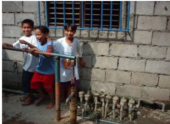
Meters replacing hand-pump, Manila, Philippines
