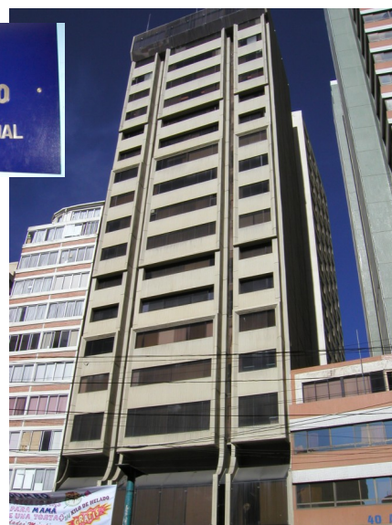
SISAB office on one floor of building
