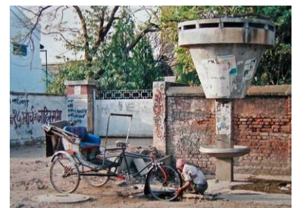
Figure 3.7. Communal yard connections with raised or ground tank
