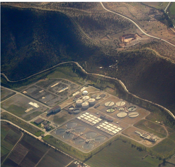
Above: New waste water treatment plant, Santiago
