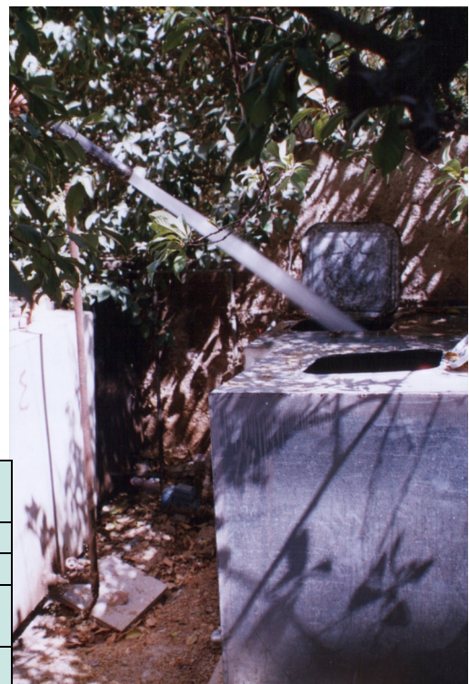
Below: Storage tank filling; note the high risk of contamination as dust and dead leaves are swept into the tank
