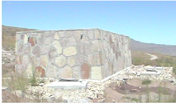
Figure 24: Typical RWS Reservoir in Natural Stone
