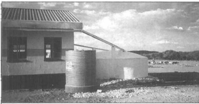
A new 46m 3 ferrocement roof tank at a primary school near Kanye.
