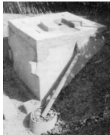
Urine diverted from squat plate to a soak pit. Senegal (photo: Del Porto & Steinfeld, 1999)
