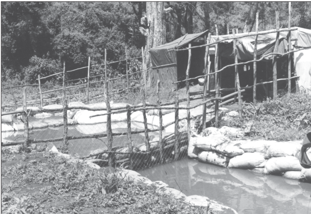
Above: Lake abstraction, Rwanda Below: Stream abstraction, Nyamirangwe Camp, Eastern Zaire
