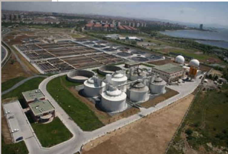
Ataköy Advanced Biological Wastewater Treatment Plant
