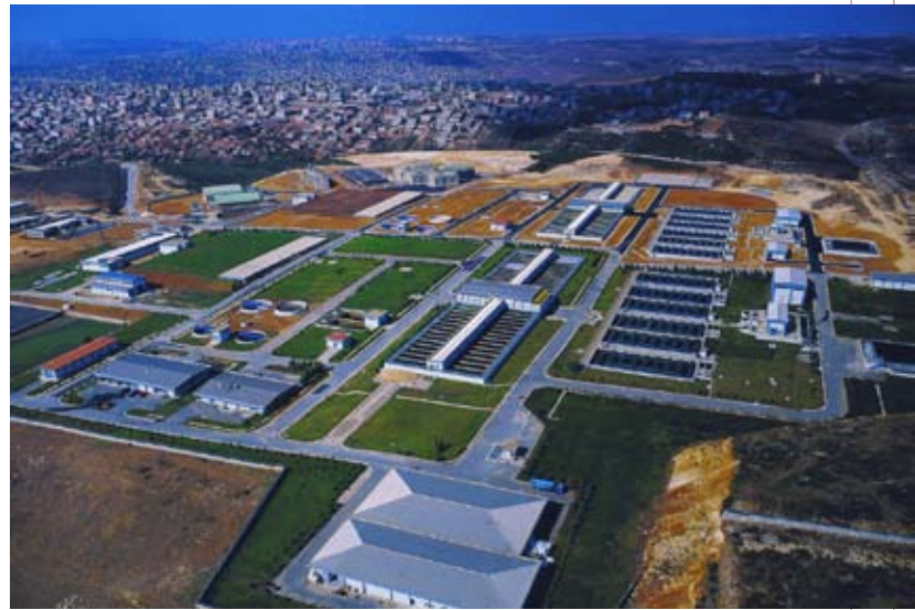
Ikitelli Drinking Water Treatment Plant
