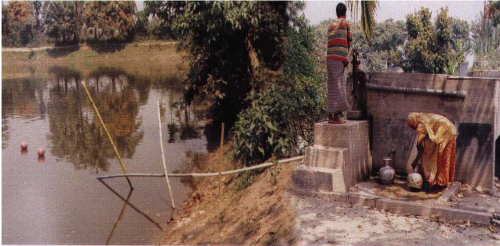
Figure 7. Pond sand filter
