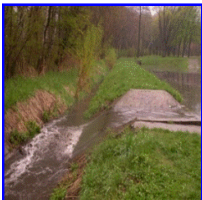
Pond improvement by Sokolowka River
