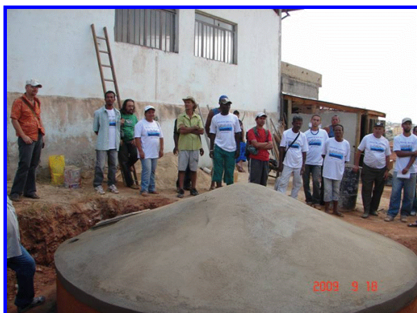
Installing a tank for rainwater harvesting
