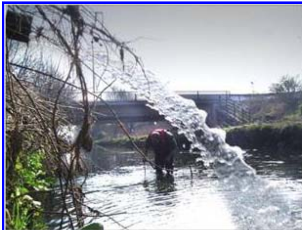
Groundwater pumping test by River Tame
