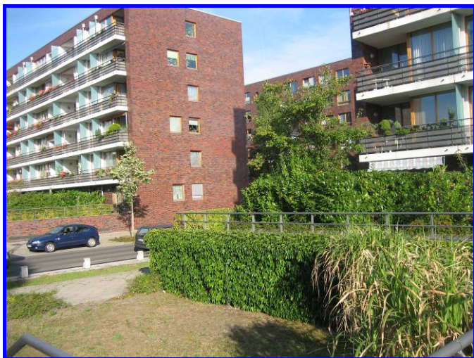
Green roofs and walls in Berlin
