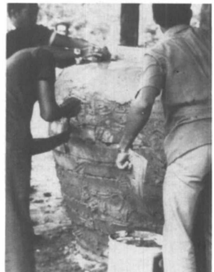
Applying mud to the outside of the bricks Photo: ATA
