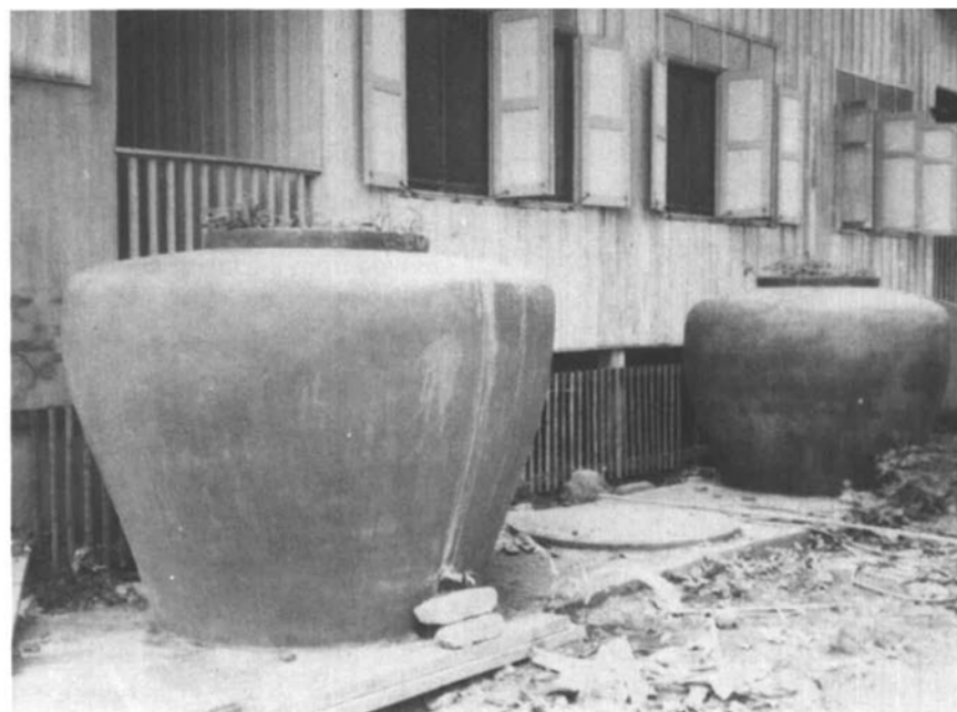
After finishing and hardening, two of the characteristically-shaped jars in place
