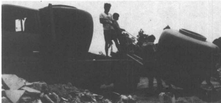
Loading for shipment from the factory yard
