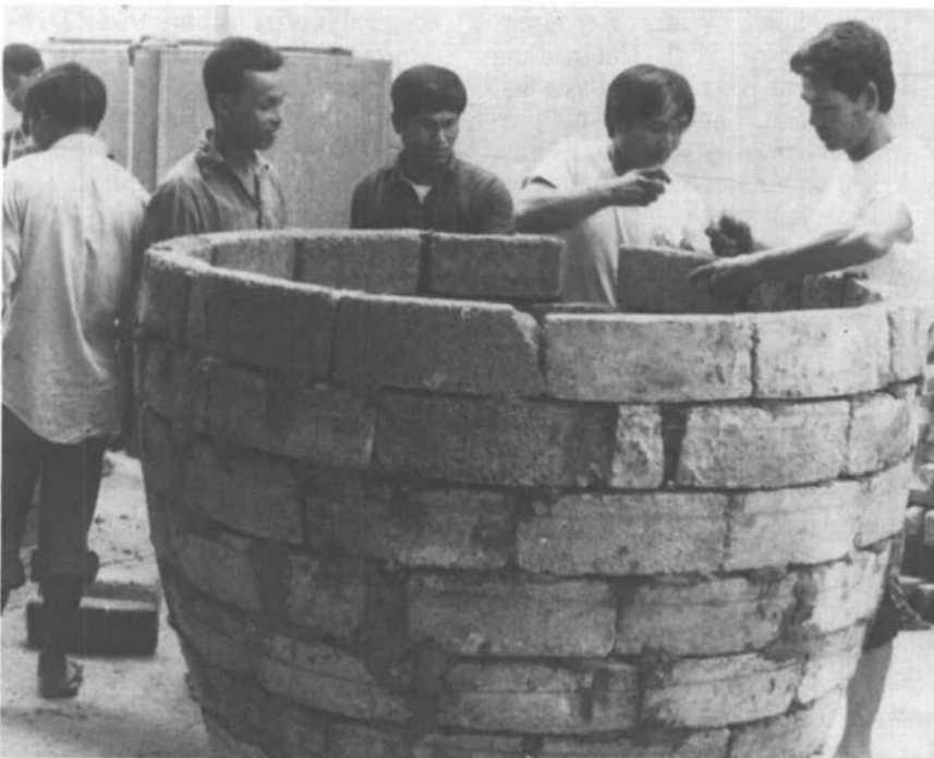
Assembling the form from bricks and mud 'mortar' Photo: Iodine and Clean Water Project
