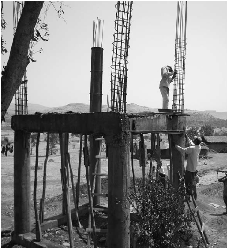
Figure 11.6 Construction of the 26,000 liter overhead tank
