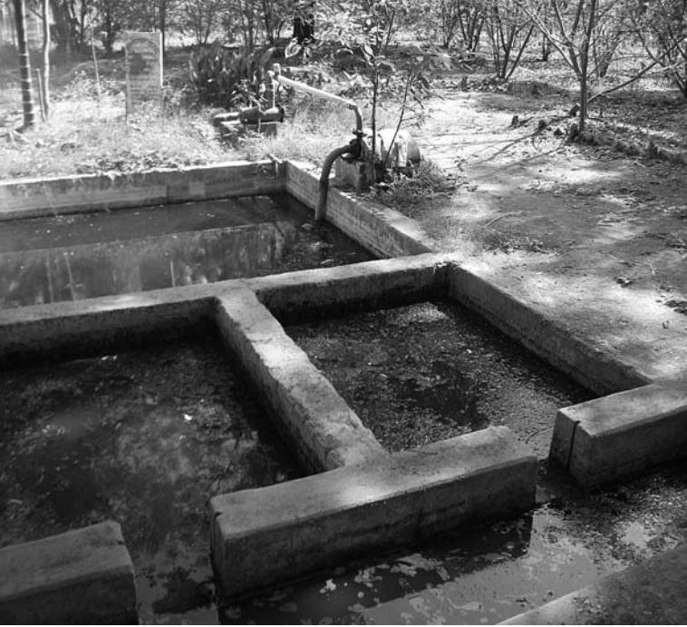
Figure 10.3 Filtration of village wastewater
