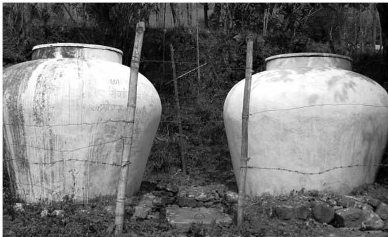
Figure 3.4 Two 3,000 liter Thai jar storage tanks
