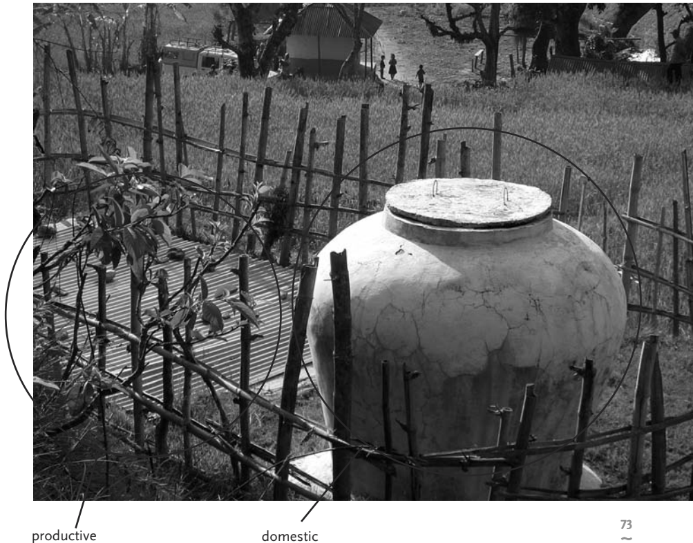
Figure 4.4 Two storage tanks for Senapuk MUS system – domestic with productive overflow Photograph by Monique Mikhail.
