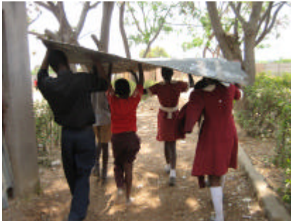
The hessian impregnated roof panel being taken to the toilet. It is laid over the roof frame and secured with wire.
