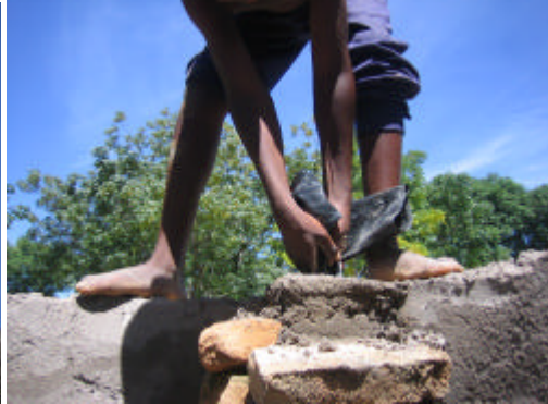
The cement mortar is allowed to cure overnight. The pipe is then removed with a twisting motion and completely removed from the toilet. Next the plastic sheet is twisted and pulled out of the cement plaster tube.
