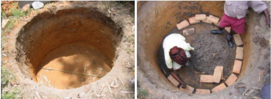
In this case the pit was dug 1.5m across and 1m deep. A mix of one part cement and 15 parts pit sand was used to make the cement mortar.
