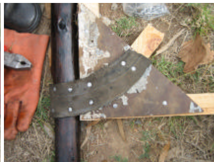
Attaching the door to a treated gum poles with rubber hinges
