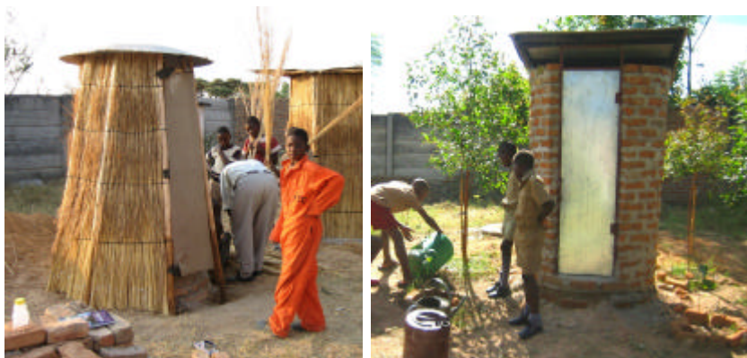
The original pole and grass structure and the upgraded brick structure
