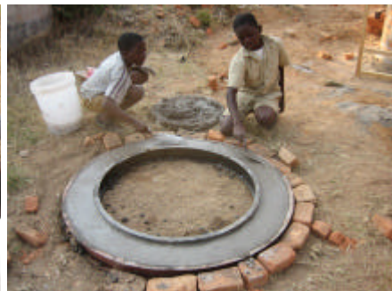
The remaining concrete is added and levelled off
