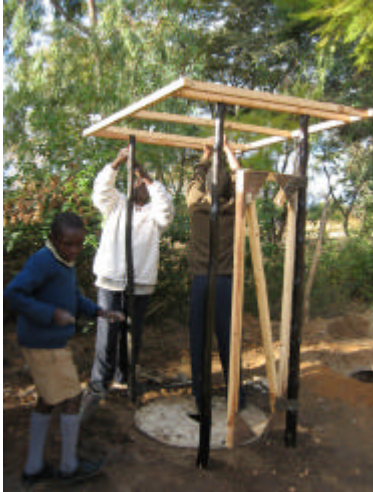
Attaching the frame to the simple treated gum poles structure. And adding the cement filled hessian sheet to the frame.
