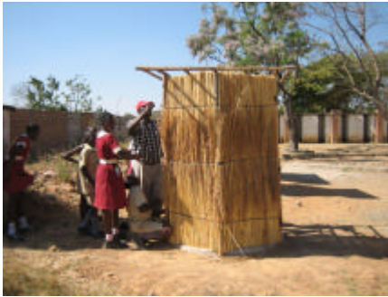
The grass structure being built. A hessian sheet was added as a door panel. This can be coated with cement slurry to make stronger. Also heavy duty shade cloth can be used or thin plywood.
