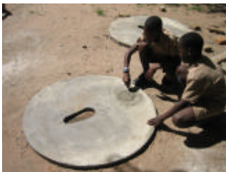
1.2m slab with vent hole filled in (temporarily) or with concrete cover.
