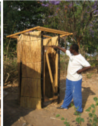
Bundles of grass are built up as walls for this toilet.
