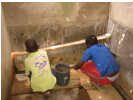
The PVC pipe is then mounted within the urinal and is supported by short brick columns. The pipes slopes downwards slightly allowing urine to flow towards the tank. The pipe should fit neatly against the urinal wall.
