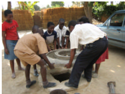
After a week of curing (being kept wet at all times) the apron is moved on to the existing well slab
