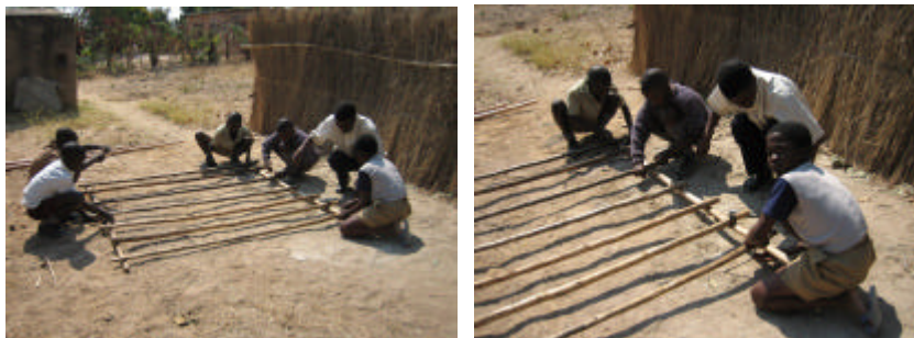
Binding the roof timbers with thatching twine
