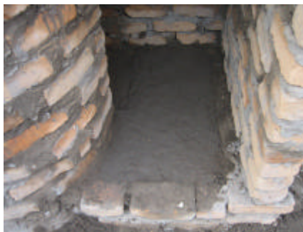
Some cement mortar is then laid on the soil placed
