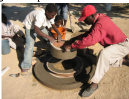
An extension to the apron is made on one side to allow water to flow off into the water run-off channel.
