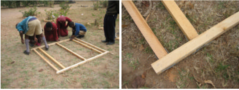
Making the roof frame
