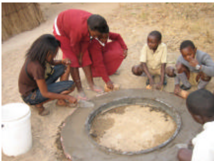
The remaining concrete is added and levelled off
