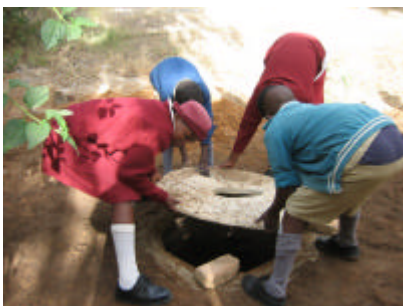
The slab is added to one of the ring beams.
