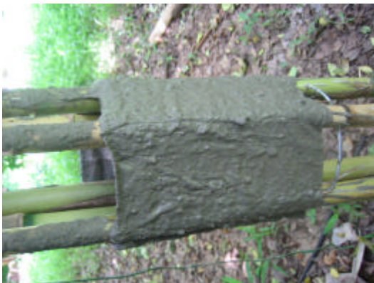
A section of the cloth is coated in a strong cement and sand slurry to demonstrate the method. The full length pipe completed.
