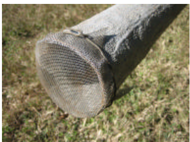
Attaching the fly screen to the vent pipe
