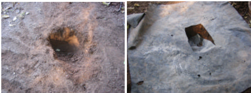
A hole is dug in the ground and a sheet of plastic is laid over it with a hole in the middle.
