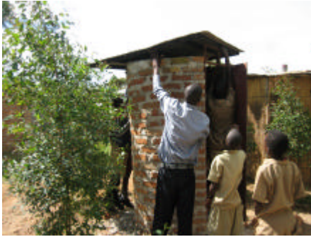
The roof is then mounted on the toilet and wired in place.
