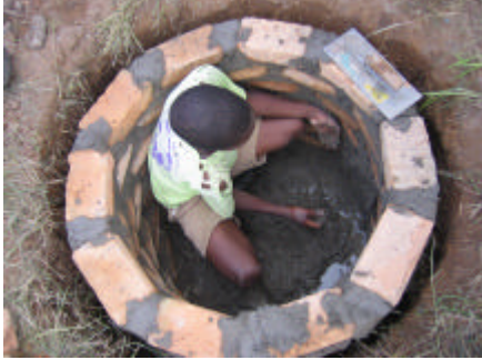
The tank is plastered from within using a strong cement and pit sand mixture.
