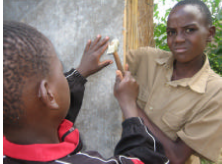
Using small nails to attach the hessian cement panel to the door frame
