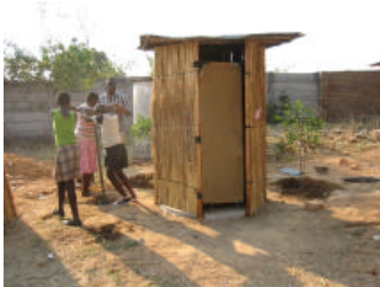
The completed toilet is surrounded by gum trees placed in holes drilled by a large earth auger (see detail in other manuals). The A hessian cement vent pipe has been added and the completed unit inspected by health officials.
