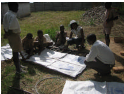
The roof frame was then made in small poles being wired together and sheets cut from plastic sacks attached with thin wire.
