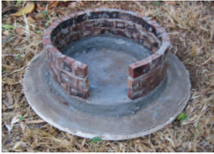
The low brick vault wall has been built on a ring beam. A second ring beam has been fitted on the brickwork and vault access door added.
