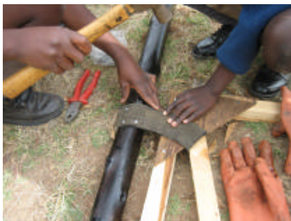
Pupils attaching the rubber hinges to the door frame and supporting pole.
