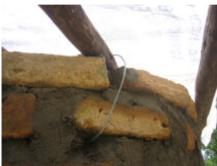
The roof timbers are secured with wire which passes through the brickwork and over the roof poles.
