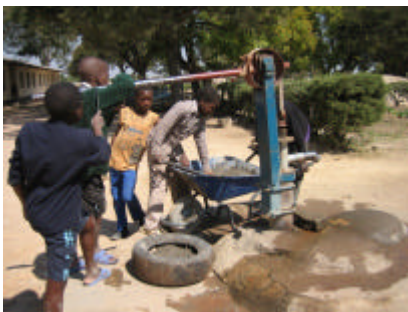
Pupils making the rubber buffer anchor and also improving the pump apron where the water is collected in buckets.
