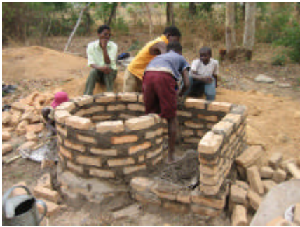
The brickwork continues upwards
