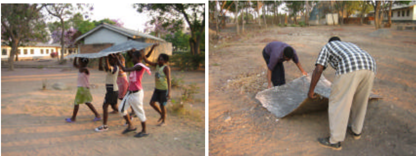
Carrying the roof sheet to the toilet.
