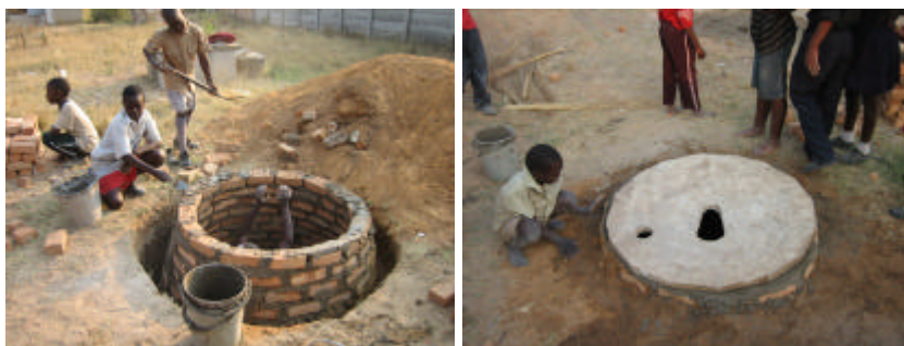
The original pit and slab
