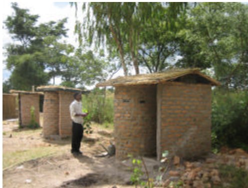
Roof in position
