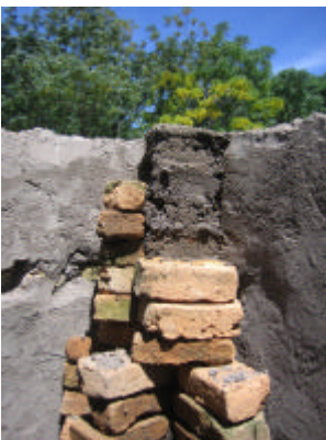
The bricks are then removed from the plaster pipe
