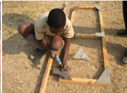
Pupils attaching the rubber hinges to the door frame and supporting pole.
