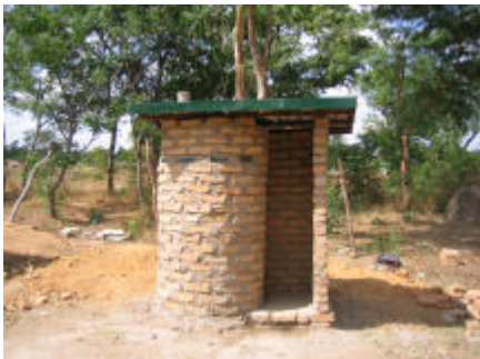
The final structure looks smart. The pipe is fitted with a fly screen.
