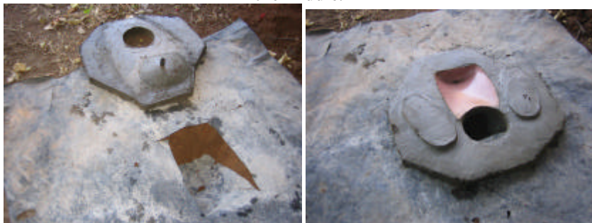
The slab can then be placed over the plastic sheet so the urine pipe enters the hole.
