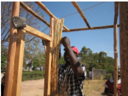
3 wires are attached tightly around the poles on to which the grass will be attached. Using thatching rope the grass is added to the structure.
