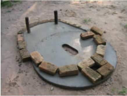
The finished toilet floor before mortaring the bricks in place. The arrangement of the brick pipe around the 140mm diameter hole.
