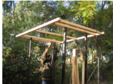
A roof frame wired together and wired to superstructure poles
