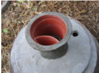
The slab has been added and hole enlarged to suit the urine diverting device used. A miniature urine diverting pedestal is shown.
