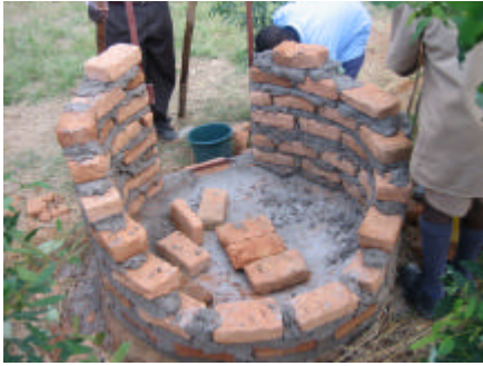
The brick work rising up. Right photo shows steel sprags welded to the frame. These are embedded in the cement mortar used to bon the bricks together.
