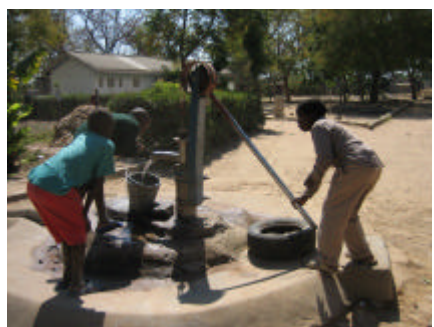
Pupils making a rubber buffer for the steel handle at the rear of the pump
