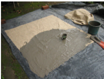
The cement paint is thoroughly applied to the first sheet using rubber gloves.
