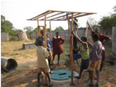
The roof frame is fitted and nailed to each of the upright poles
