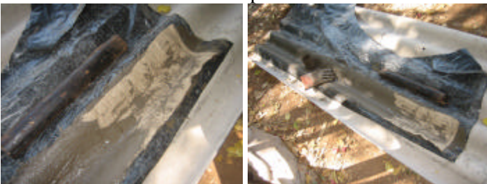
The hessian cement water run-off channel 1.5m long
