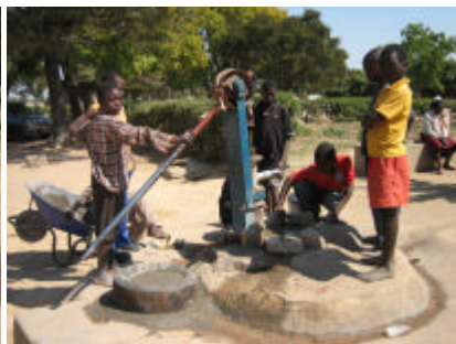
Pupils making the rubber buffer anchor and also improving the pump apron where the water is collected in buckets.
