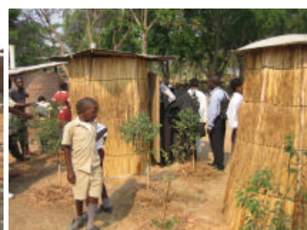
The completed toilet is surrounded by gum trees placed in holes drilled by a large earth auger (see detail in other manuals). The A hessian cement vent pipe has been added and the completed unit inspected by health officials.
