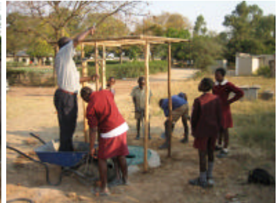
The roof frame is fitted and nailed to each of the upright poles
