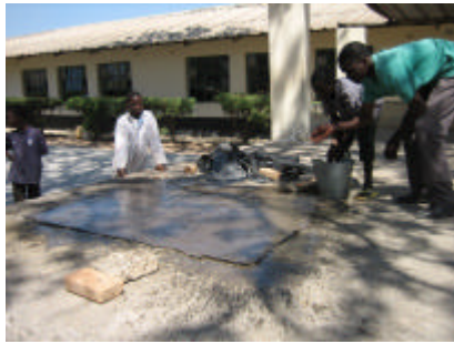
Once fully thatched a cement impregnated roof sheet is made on flat ground and left to cure for 3 days under plastic sheet.
