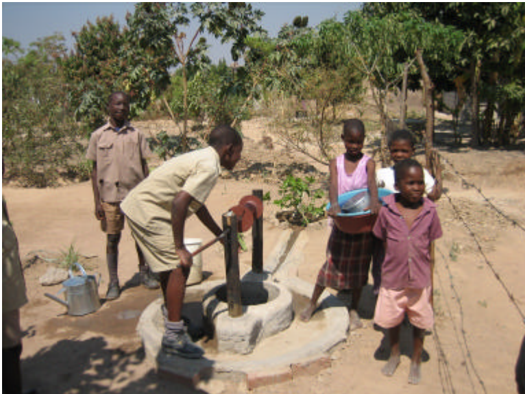
The completed well. A fitting tin lid is prepared to make a well cover. Diluted urine can be used to fertilise the tree. 2 litres of urine diluted in a 10 or 12 litre watering can or bucket of water can be added once a week. As the tree grows larger extra manure or compost can be added to the soil surrounding the tree. The advantage of planting a tree at the end of the well run-off is that the tree will receive water regularly.
