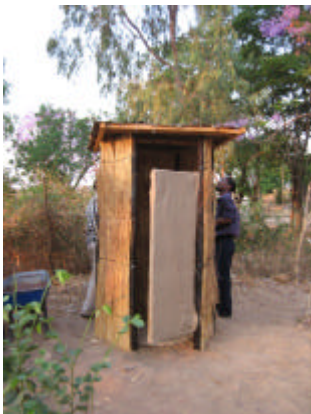
The roof sheet is attached to the roof sheet using small nails. The roof frame can either be nailed or wired to the supporting poles.
