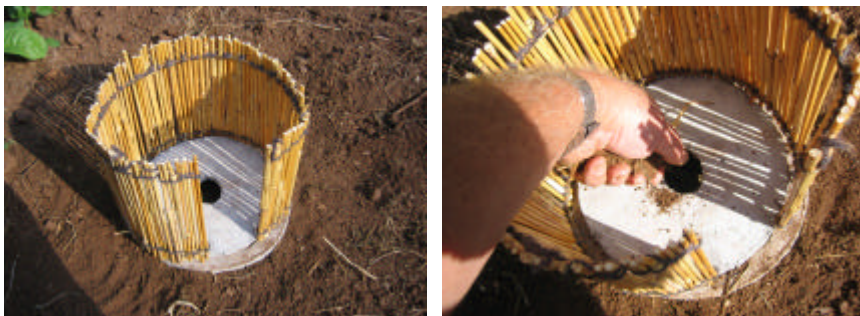
The simple structure is now fitted and the Arborloo put to use
