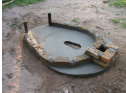
The bricks are laid in the mortar so they join up with the door posts in a gentle curve (horseshoe shape). A second course of bricks is laid for the vent pipe. The brick walls and pipe are then extended upwards so the final height of the wall is about 1.8m and the vent 2.3m.
