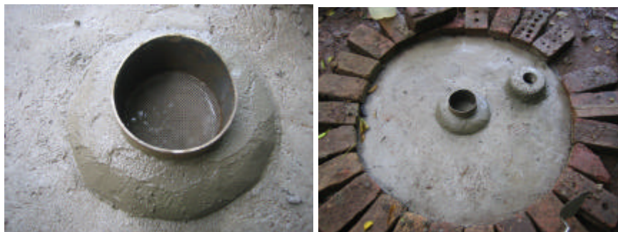
Central hole of upper tank slab with stainless steel screen and also the concrete plate made to hold the 50mm steel pipe socket in which the hand pump (Blair Pump) is screwed.
