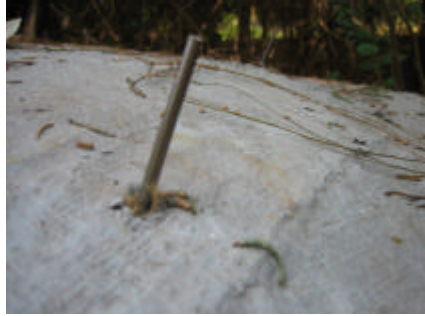
View of the nails hammered into the poles before and after the hessian cement roof was fitted.
