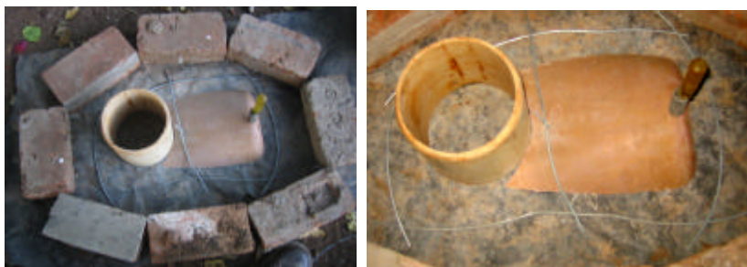
Cut “urine catcher” placed within a brick mould together with a squat hole mould. Design by Annie Shangwa.
