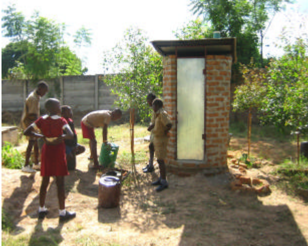
The completed toilet.
