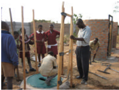
The door frame is fitted to the main “king post” with rubber hinges. Meanwhile a timber roof frame is made up to fit over the 6 upright poles.
