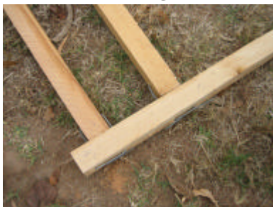
A roof frame wired together and wired to superstructure poles
