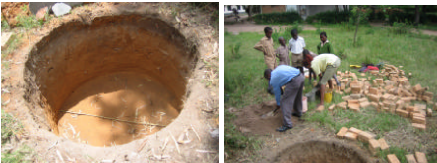
Dig hole and assemble bricks
