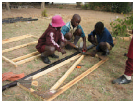
Attaching the door to a treated gum poles with rubber hinges
