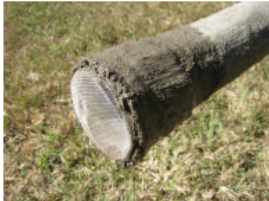
Attaching the fly screen to the vent pipe
