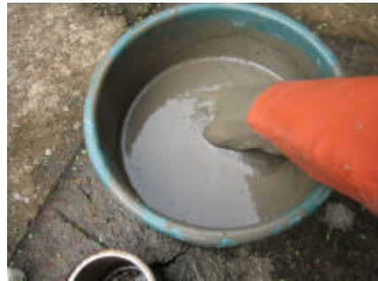
Hessian sheet laid over plastic sheet. Stirring the cement paint mix.
