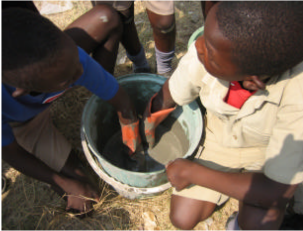
The cement mix is stirred thoroughly using rubber gloves.
