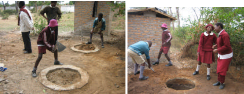
Lay 2 ring beams and dig 2 pits inside
