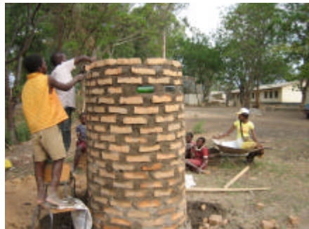
Photo showing glass bottles in wall. The full height of the superstructure is about 19 courses of bricks.
