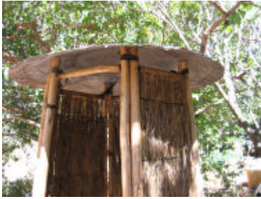
A domed cement impregnated hessian roof is added on top and can be wired in position for security.
