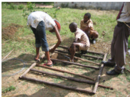
The roof frame was then made in small poles being wired together and sheets cut from plastic sacks attached with thin wire.
