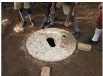
Slab fitted ready for toilet house
