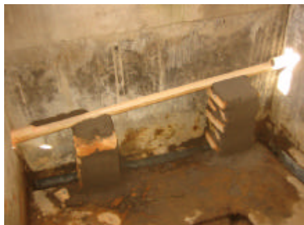
The PVC pipe is then mounted within the urinal and is supported by short brick columns. The pipes slopes downwards slightly allowing urine to flow towards the tank. The pipe should fit neatly against the urinal wall.
