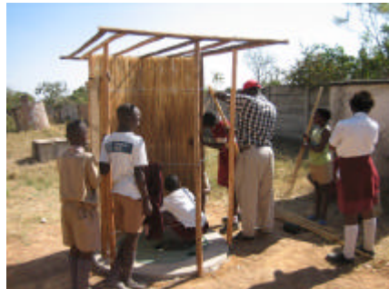
3 wires are attached tightly around the poles on to which the grass will be attached. Using thatching rope the grass is added to the structure.
