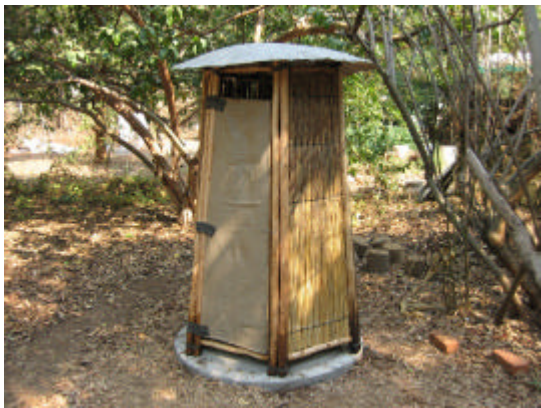
A suitably sized door panel is made and fitted the main post with rubber hinges. A hessian door covering is attached to provide privacy.
