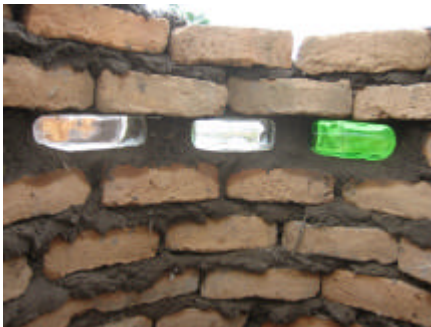
Photo showing glass bottles in wall. The full height of the superstructure is about 19 courses of bricks.
