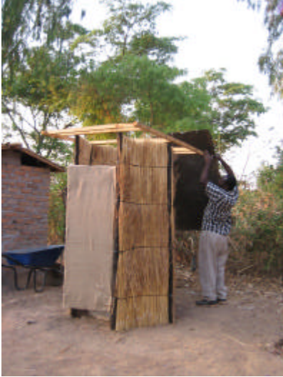
The roof sheet is added to the roof frame and secured with small 25mm nails
