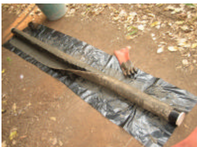
Stages of apply the cement paint
