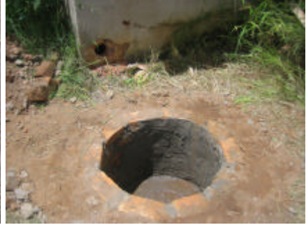
The tank is plastered from within using a strong cement and pit sand mixture.
