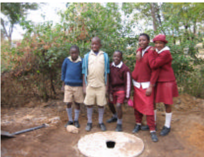
Slab fitted ready for toilet house
