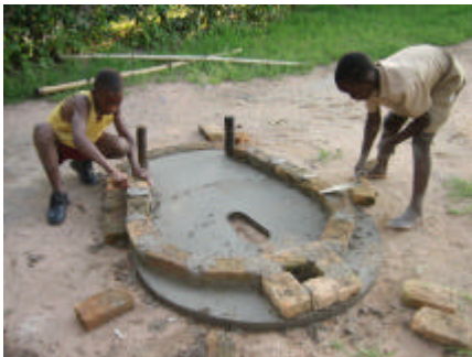
The bricks are laid in the mortar so they join up with the door posts in a gentle curve (horseshoe shape). A second course of bricks is laid for the vent pipe. The brick walls and pipe are then extended upwards so the final height of the wall is about 1.8m and the vent 2.3m.
