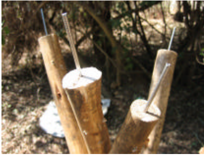
View of the nails hammered into the poles before and after the hessian cement roof was fitted.
