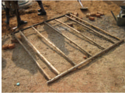
The door frame is fitted to the main “king post” with rubber hinges. Meanwhile a timber roof frame is made up to fit over the 6 upright poles.
