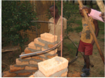
The brick work rising up. Right photo shows steel sprags welded to the frame. These are embedded in the cement mortar used to bon the bricks together.
