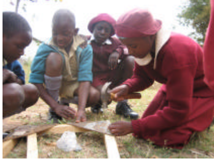
Pupils putting together the door frame with triangular pieces of plywood and nails.
