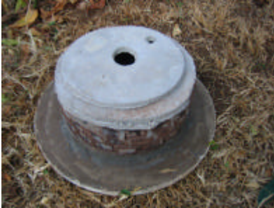
The slab has been added and hole enlarged to suit the urine diverting device used. A miniature urine diverting pedestal is shown.
