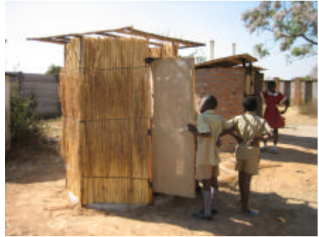
The grass structure being built. A hessian sheet was added as a door panel. This can be coated with cement slurry to make stronger. Also heavy duty shade cloth can be used or thin plywood.
