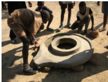
After a week of curing (being kept wet at all times) the apron is moved on to the existing well slab
