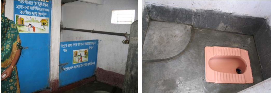
Sanitation blocks in Dhaka Slums, ASEH 2006: Child friendly facilities and washing platform for menstrual rags
