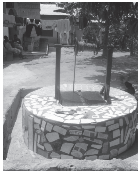
Photograph 2. Hand-dug well with pulley system
