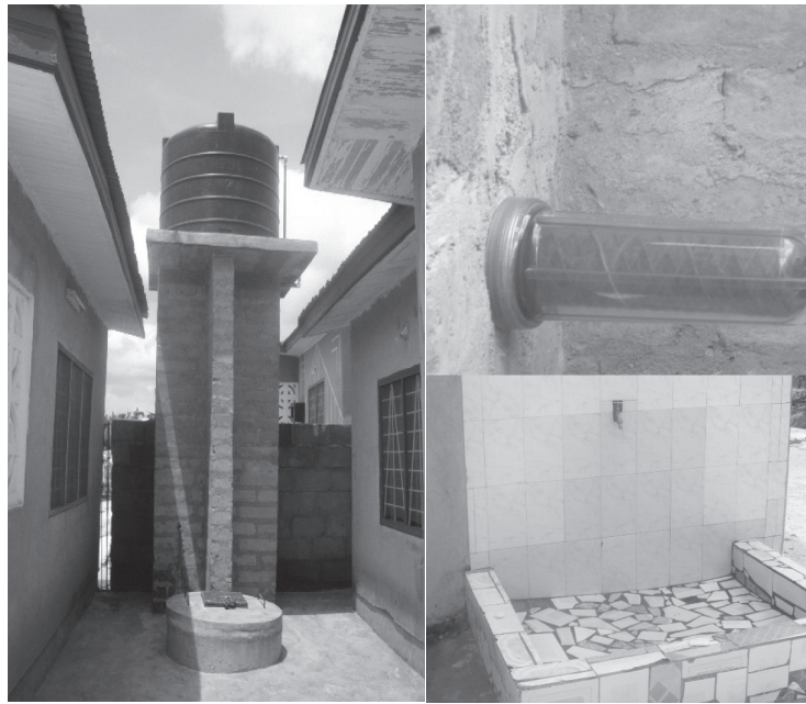
Photograph 3. Mechanised hand-dug well with pump, elevated storage tank, filter and a tap
