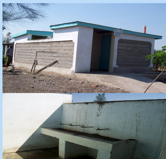
Figure 1. Exterior and taps of KESSP-design latrine/washroom facility at Kamunda Primary, constructed by Water.org.
