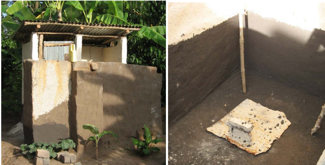
Upgraded latrine in Luweero District. Total Cost (pit + structure): 115,000 Ushillings
