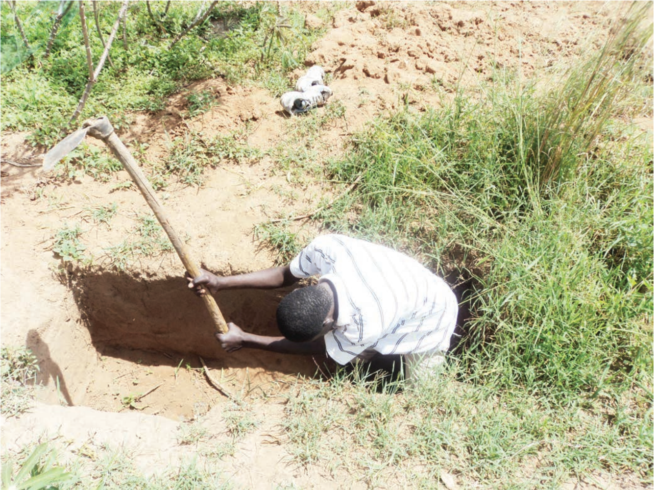
Pit digging after triggering in Atiri parish, Tororo district.
