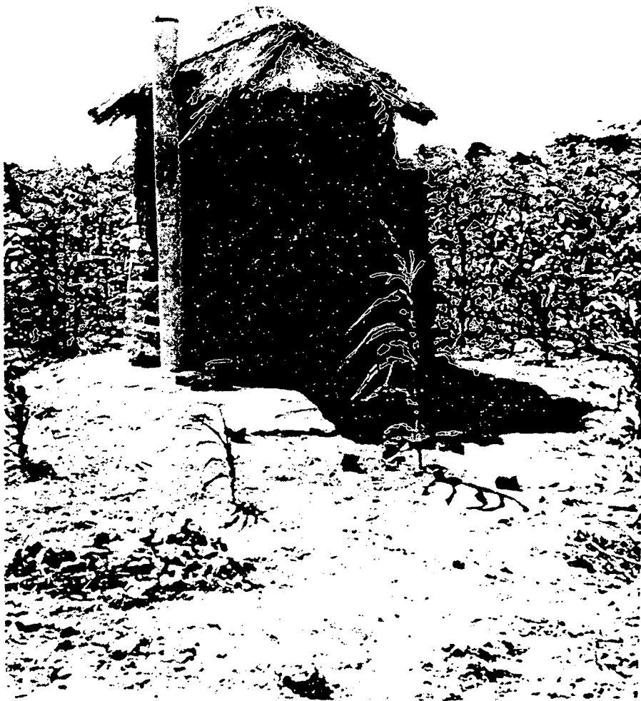
Photograph No 1 : One variety of the Zimbabwe Ventilated Improved Pit Latrine. Zimbabwe VIP options have been developed with a close regard for the social soundness of the technology, and their development is a model of socio-technical design. Particular attention was paid to the acceptability of the design in rural Zimbabwe, to local hygienic practices, and to affordability. The cheapest option retains all the public health benefits of ventilation and other aspects of the design and yet costs under US$5.
