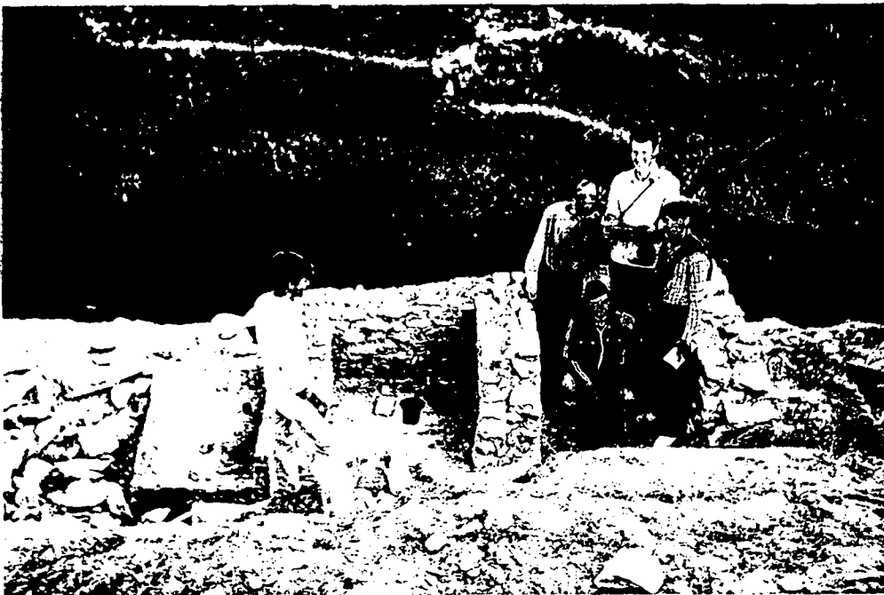
Testing the ferrocement squatting slab of a 2-unit VIP school latrine
