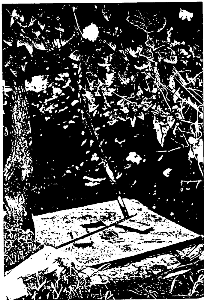
... with ferrocement squatting slab and HDP vent pipe
