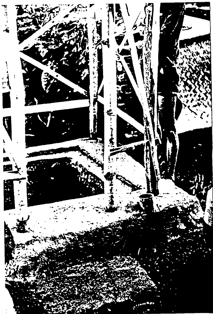
... with ferrocement squatting slab and HDP vent pipe
