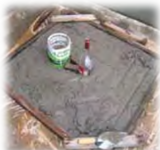
Two types of shiftable platforms; Low-cost full-cycle toilets (Photos by Jo Smet, IRC).
