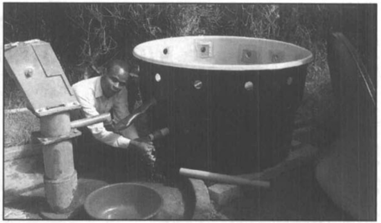
Installing the iron-removal filter in Lyontonde (above). Teaching local children about health and hygiene (left).
