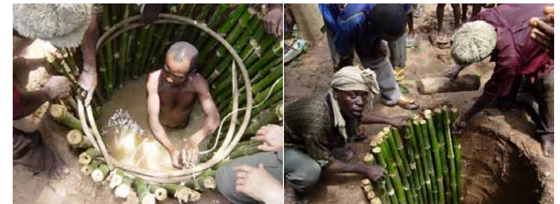
Community sanitation committee members drive bamboo rods in Obijago Community, Obi LGA (left), a softwood hoop is installed and secured with rope (right).
