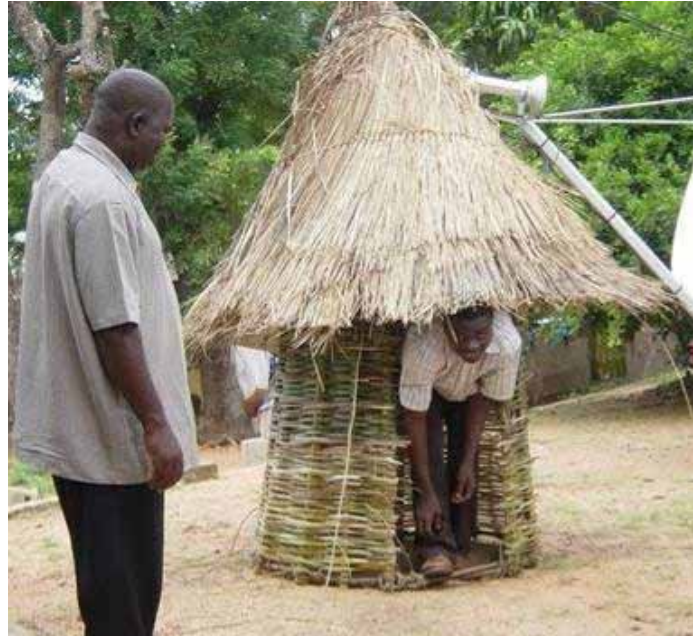
An arborloo, constructed of woven palm fronds at the WaterAid office in Makurdi.
