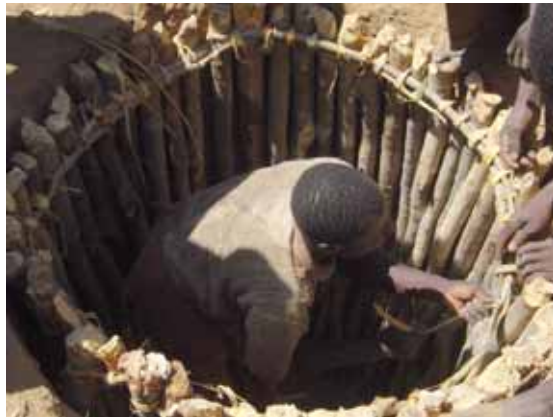
Local artisans secure a flexible hoop at the top of a hardwood pit in Balzur Community Tafawa Balewa LGA, Bauchi State (left), The cage is subsequently encased in mud treated with latrite and a collar beam is formed at the top.
