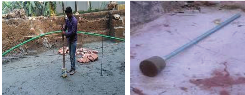
Fig-17: Manual Compaction
