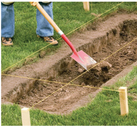
Figre-12: Trench excavation
