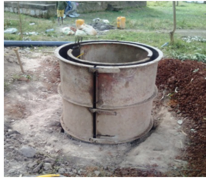
a) Concrete ring cast on pit
