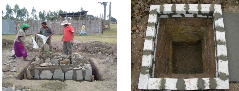
Fig-7: Under ground masonry wall construction
