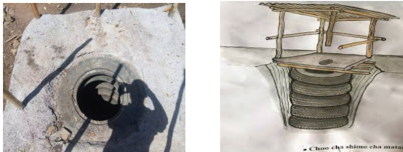
Fig-8: Used tyre pit lining.
