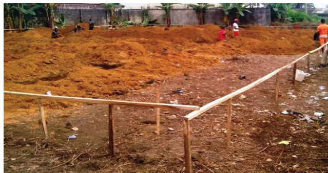
Figure-11: Excavation work
