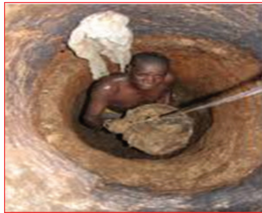
Figre-13: Circle trench excavation
