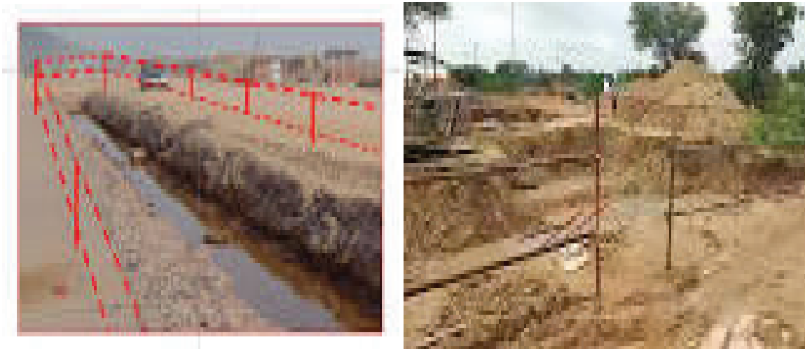
Figure-10: Barricade in excavation
