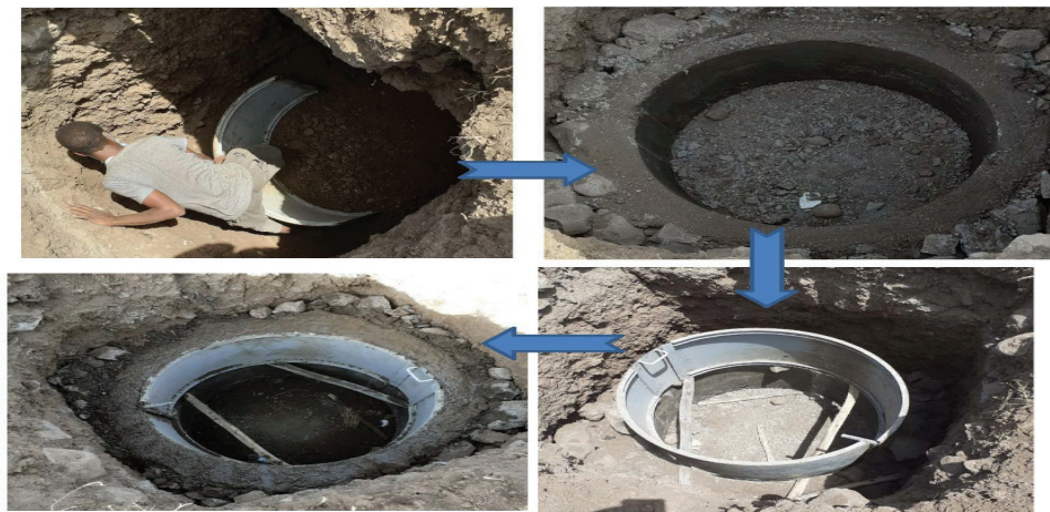
Figure-9: Cast on site inside pit.
