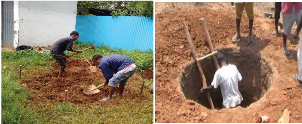
Fig-5: Circle latrine pit excavation
