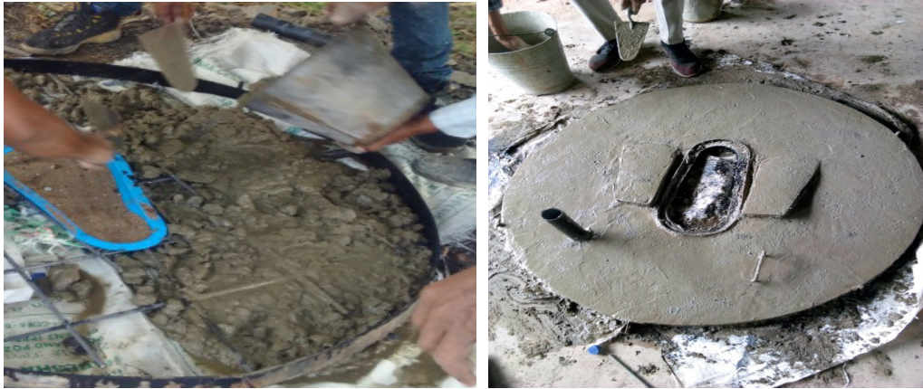
Fig. 25: Placing of concrete.
