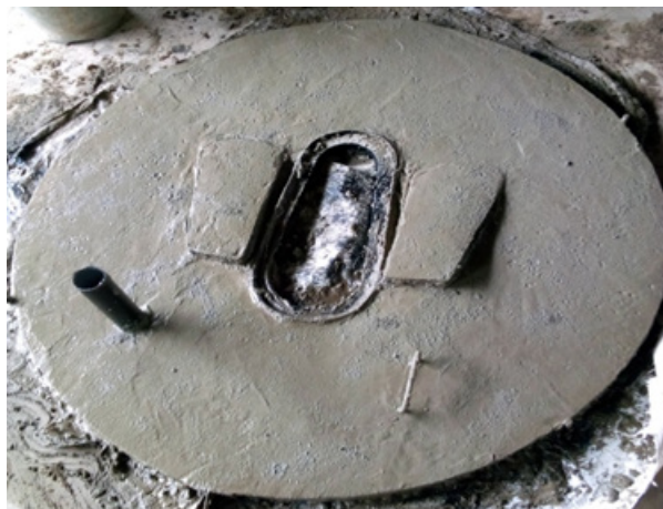
Fig. 29 circular concrete slab
