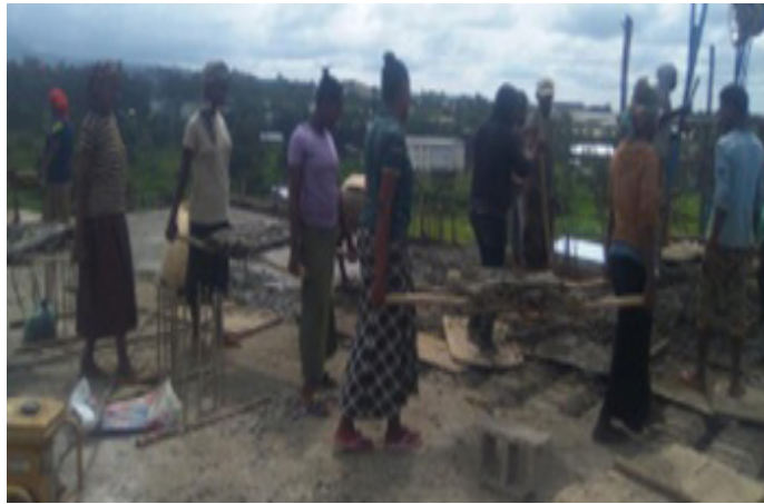
Fig. 23: Transporting of concrete.
