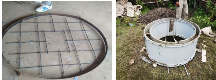
Fig.14: Steel form work/ mold
