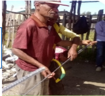
Fig-7: Cutting of rebar.
