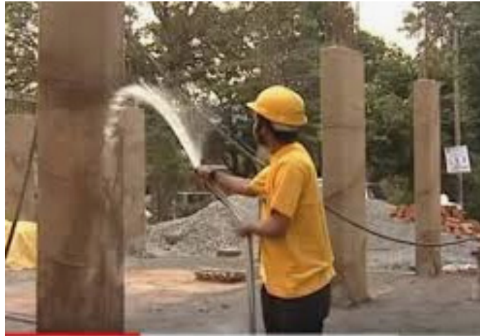
Fig. 28- Curing of concrete
