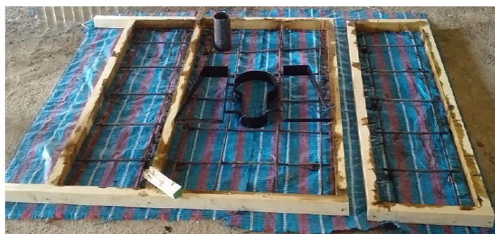
Fig. 13: Wooden form work to cast concrete slab
