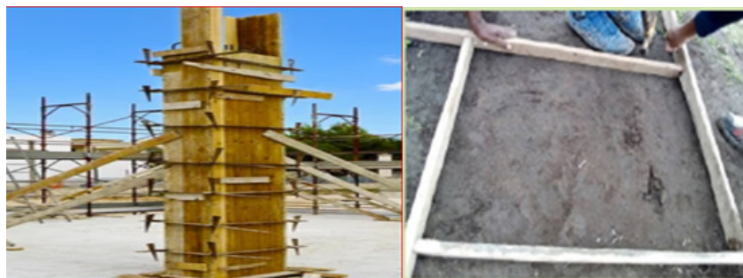
Fig-12: Form work to cast slabs and column
