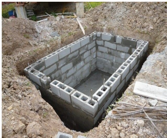
Figure.3.19. Erecting rectangular wall
