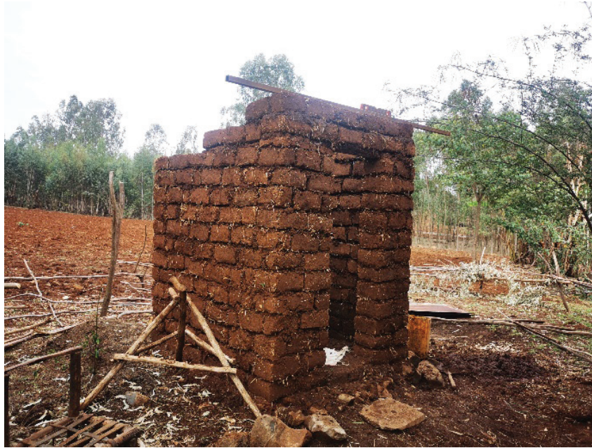
Figure: 2.2. Toilet wall construction with mud block
