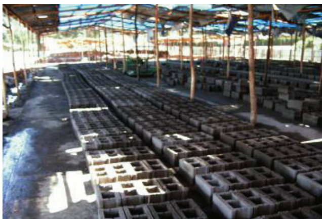
Figure-1.10. Shade for Freshly Cast Block Protection....
