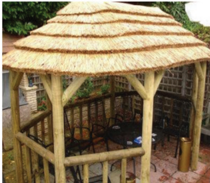
Fig.5.2. Thatch Roof
