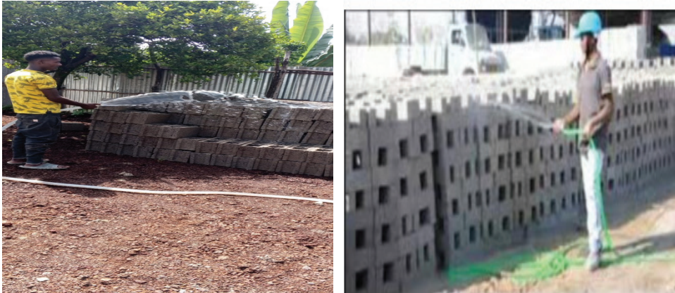
Figure: 1.11. Curing of concrete block
