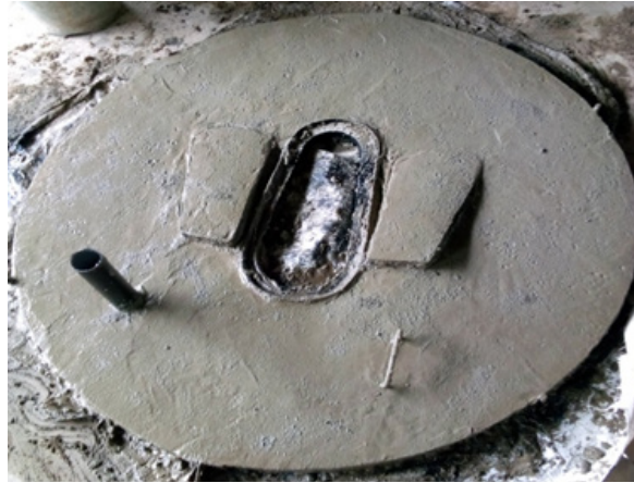
Fig. 29 circular concrete slab
