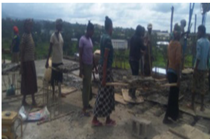
Fig. 23: Transporting of concrete.
