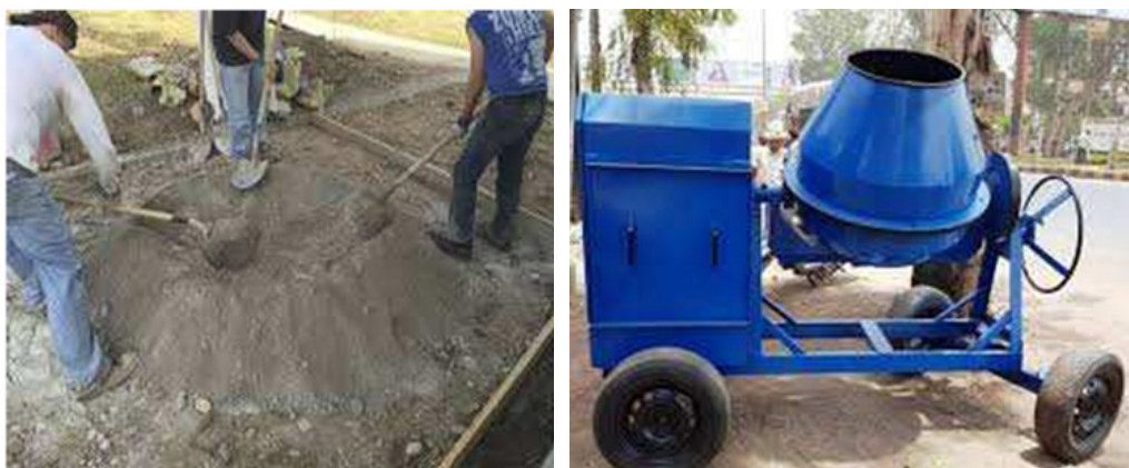
Fig-22: Hand and mechanical mix
