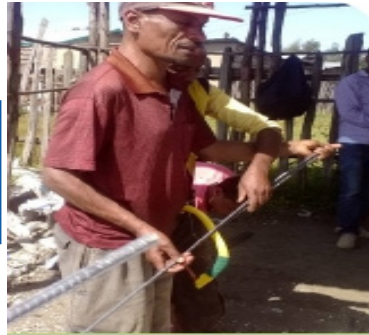
Fig-7: Cutting of rebar.
