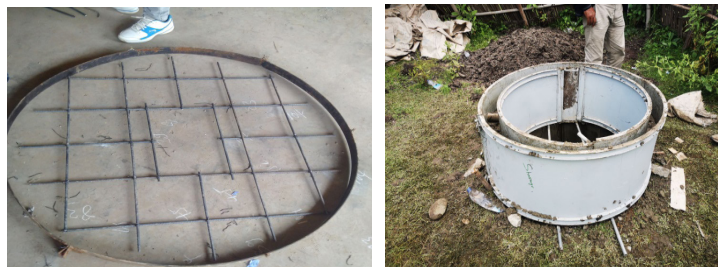
Fig.14: Steel form work/ mold
