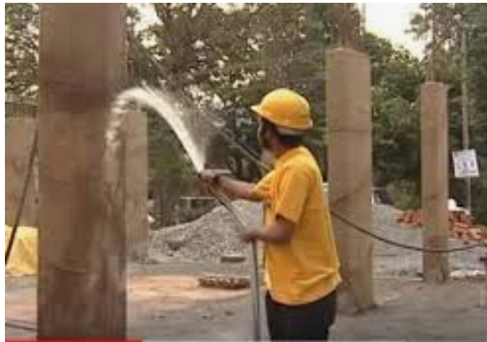
Fig. 28- Curing of concrete
