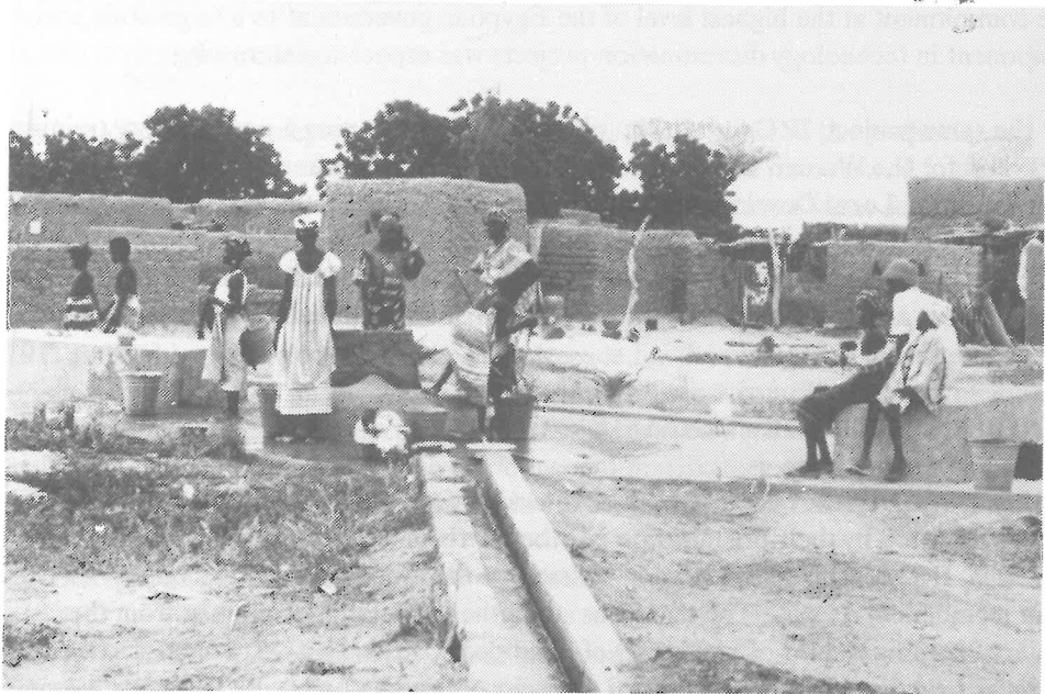
Improved well with extended slabs, drainage channel, and laundry facilities in Mali.
