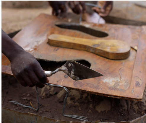
Promoters making a latrine slab, Chikompulazi village, Mzuzu, Malawi. Credit: WaterAid/Layton Thompson.
