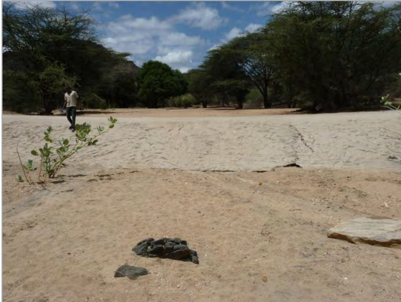
Figure 5-11: Concrete road-crossing through a riverbed, creating a sanddam
